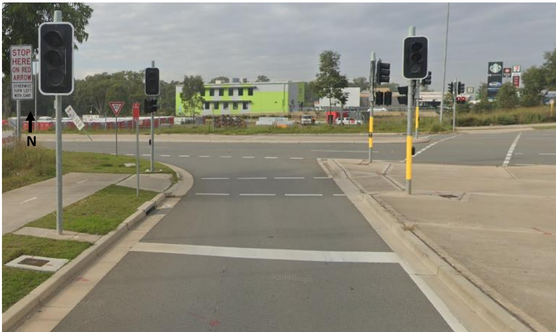
Figure 5.3 Indicative single slip lane configuration
