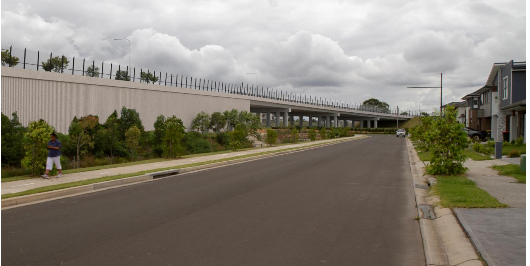
Figure 3-6: Illustration of the reinforced soil wall bridge and rail bridge looking north-east from Anson Street with indicative screen planting
