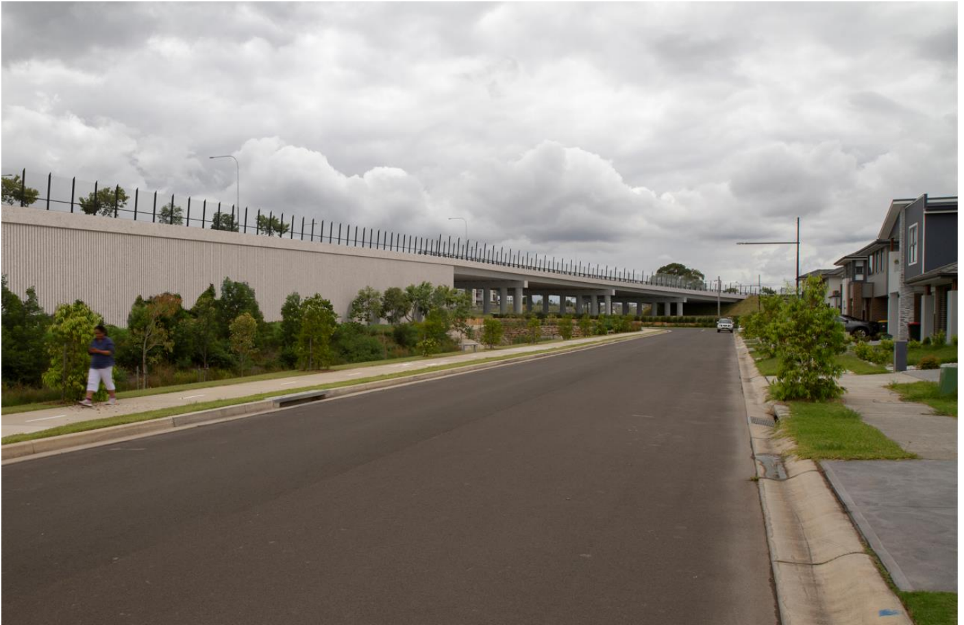
Artist's impression of the proposed reinforced soil wall, rail bridge and indicative planting, looking north-east from Anson Street.
