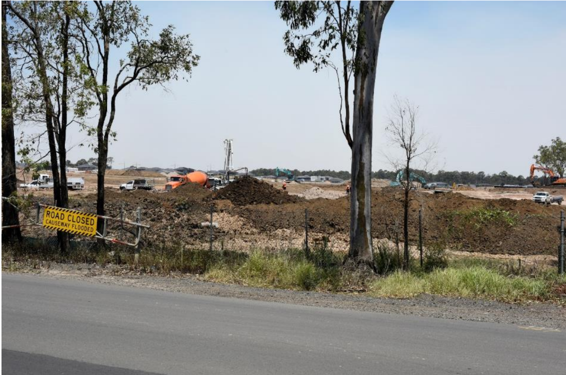
Figure 3-5 View south-east towards LCZ 4, future residential, from Townson Road
