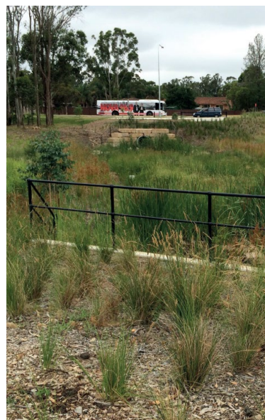
Figure 4-6 WSUD device Blacktown City Council LGA
