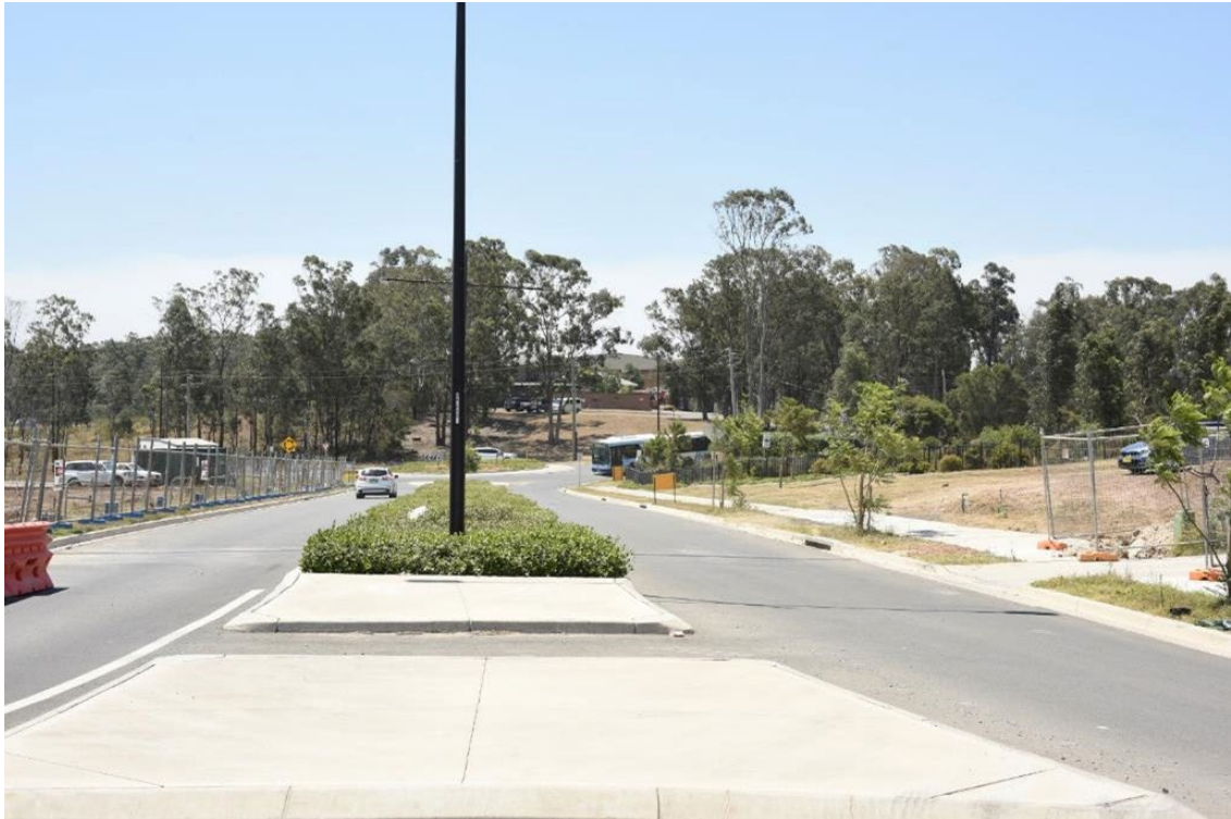
Figure 3-13 View north-west along Victory Road
