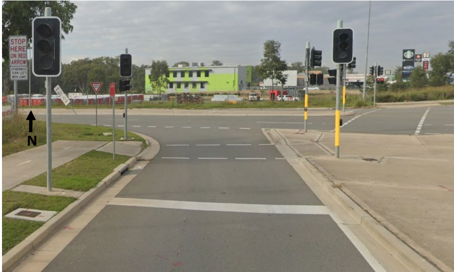
Figure 5-11 Indicative single slip lane configuration
