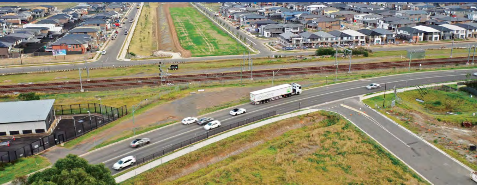
Burdekin Road looking west towards Eastern Creek
