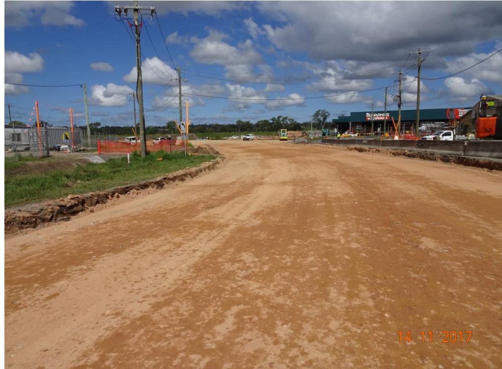
Through Street pavement construction Nov 2017
