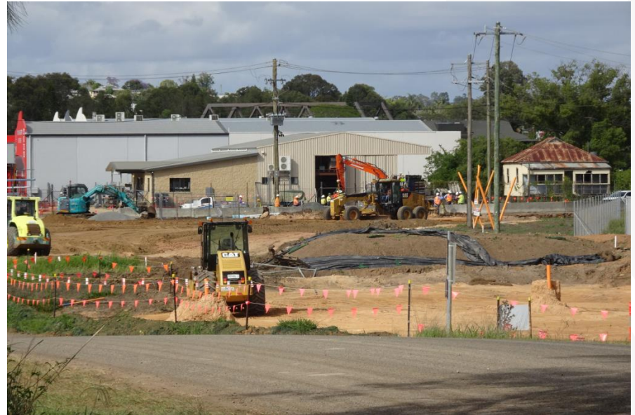
Through St road construction
