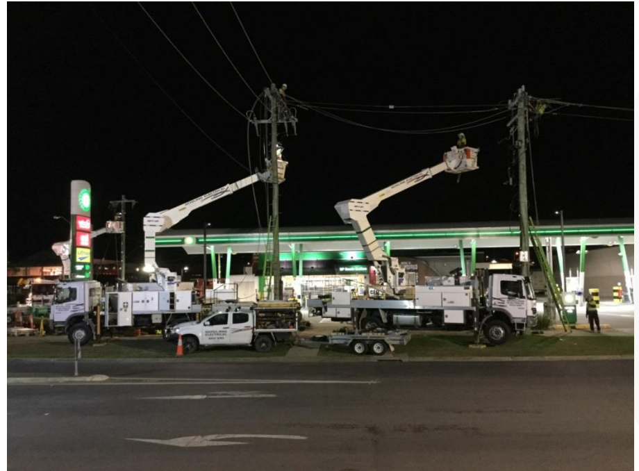
Power relocation work underway at night in South Grafton (September 2018)
