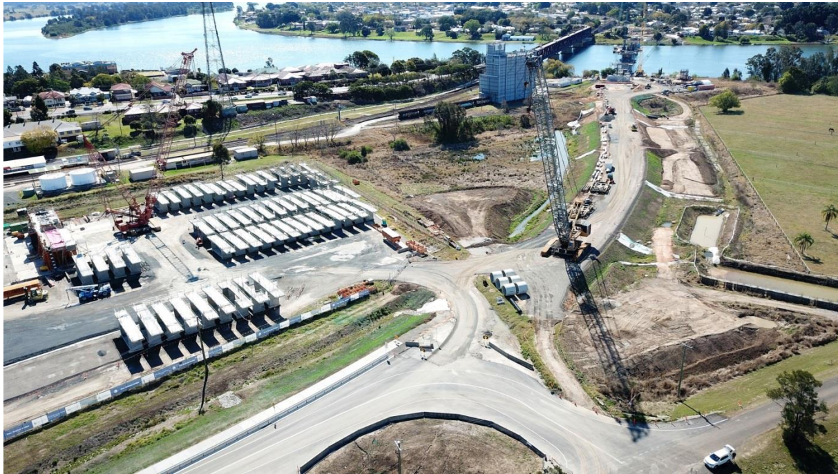
Aerial view of segments lined up in the pre-cast yard (September 2018)
