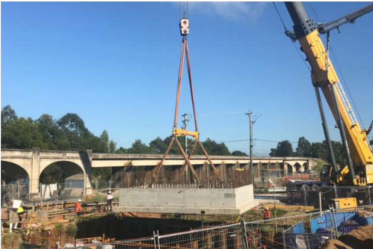
Figure 1 Pump station being lifted into place at Kent Street
