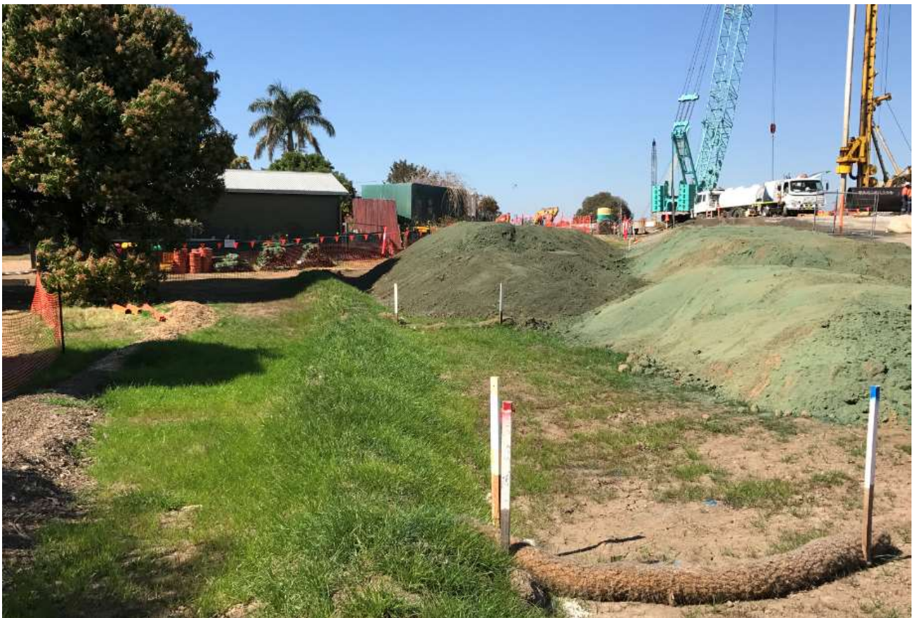
Figure 10 Grass strike and controls installed near abutment B in Grafton
