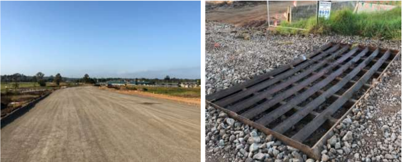
Figure 9 SMZ placed at fill 1 (left) stabilised access and egress points (right)
