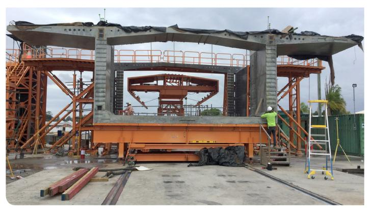
First concrete bridge segment poured at the pre-cast facility in January
