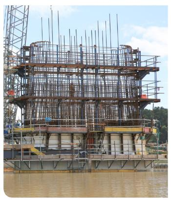
Steel reinforcement for concrete pier (March 2018)
