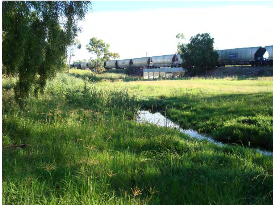
Photograph D- 3: Rail Culvert over Blackjack Creek constructed in 2011
