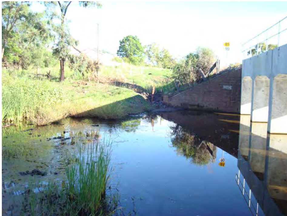
Photograph D- 5: Blackjack Creek upstream of the Rail Culvert, looking west. Note the stagnant water and reed growth.
