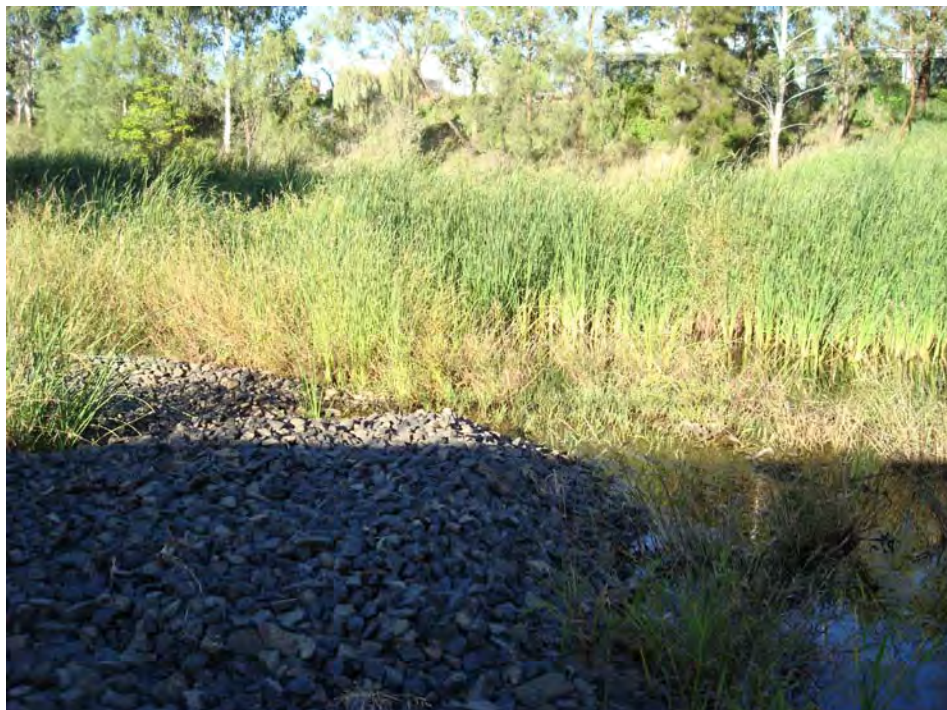
Photograph D- 6: Blackjack Creek upstream of the Rail Culvert, looking west. Note the stagnant water, reed growth and the rail ballast working platform.
