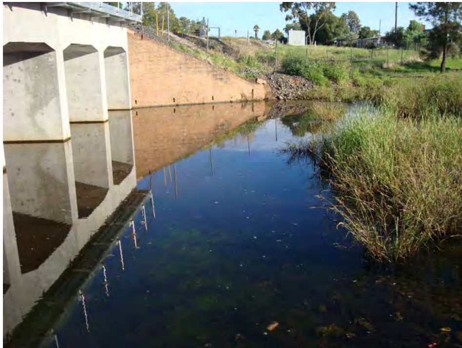
Photograph D- 7: Blackjack Downstream of Culvert
