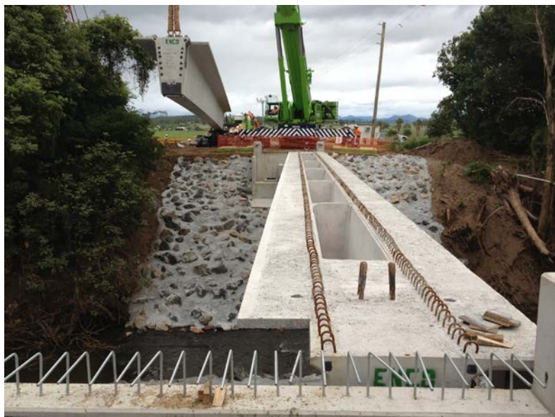
Figure 5.10: Typical super-T girder construction
