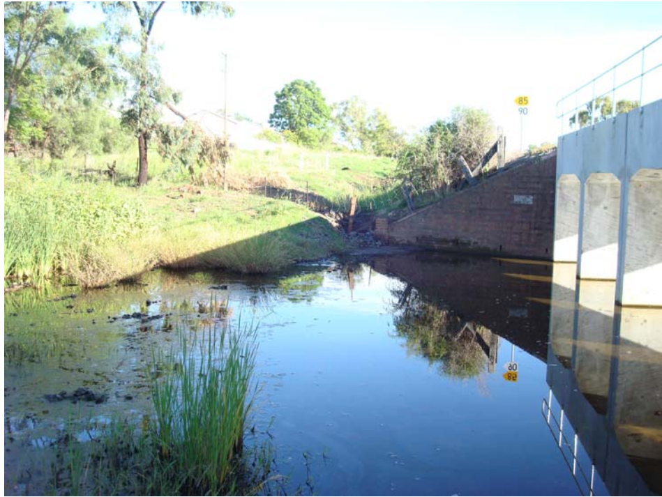
Photograph D- 5: Blackjack Creek upstream of the Rail Culvert, looking west. Note the stagnant water and reed growth.
