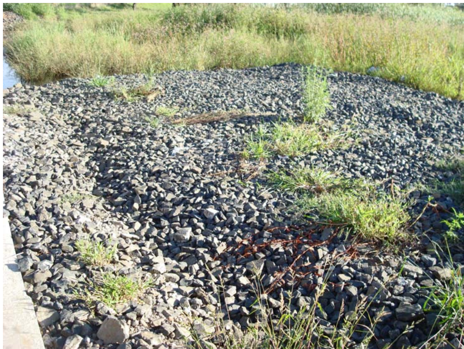
Photograph D- 8: Old working platform
