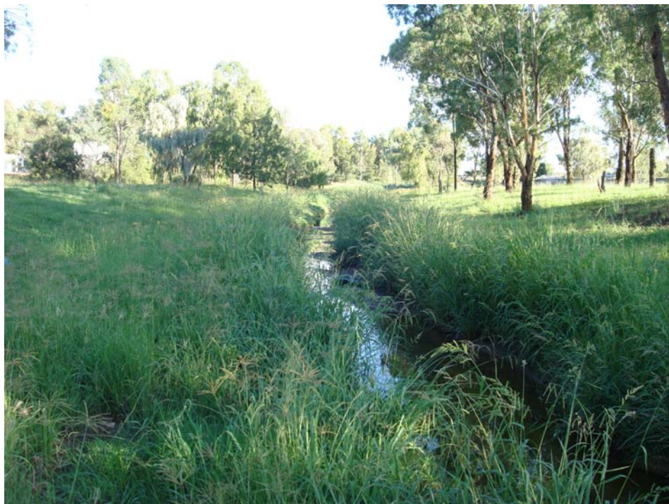
Photograph D- 2: Ashford Water Course, looking north-west from New Street. Note running water and flood debris on the right.
