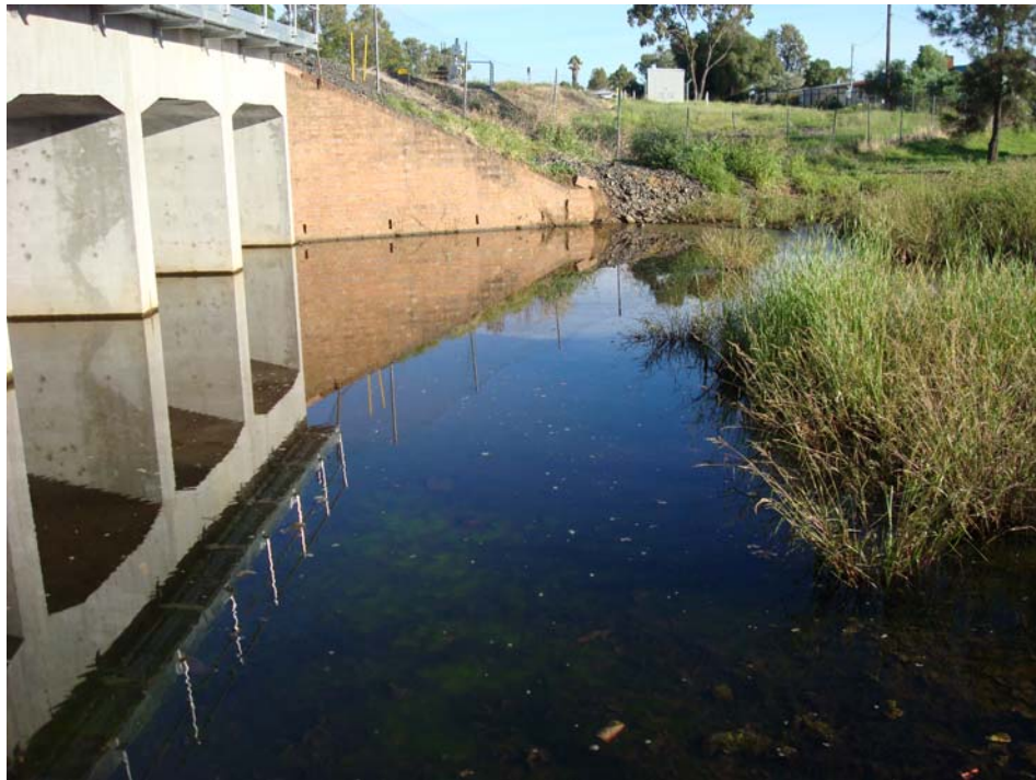
Photograph D- 7: Blackjack Downstream of Culvert
