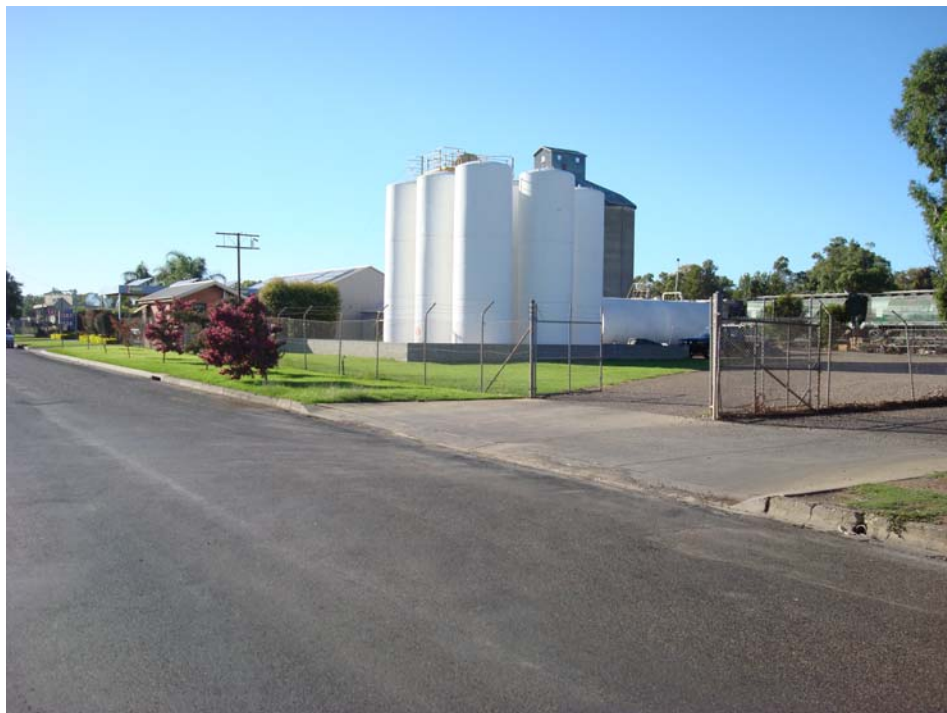
Photograph D- 10: Hope Fuel Supplies Tank Farm
