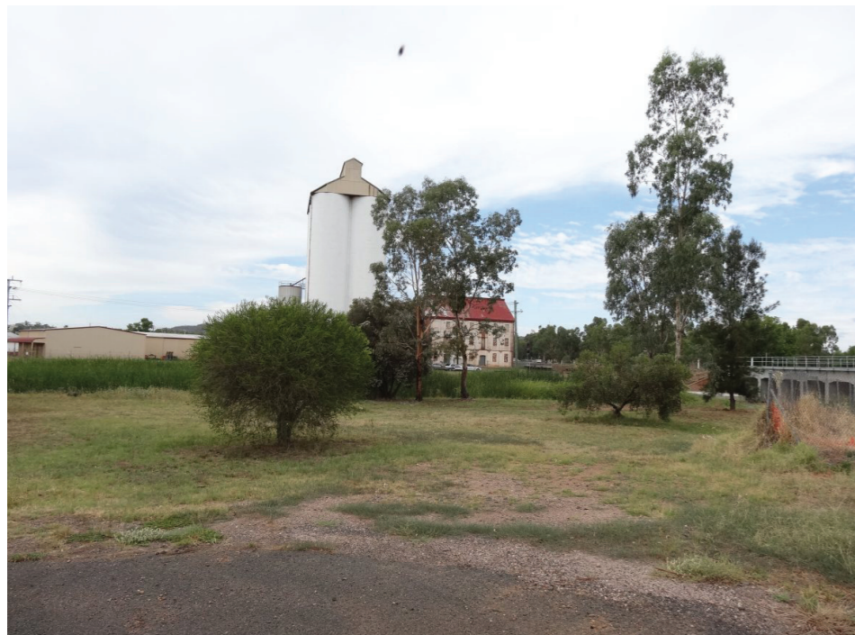
View looking south from the cul-de-sac of Stockman Close towards the Mill
