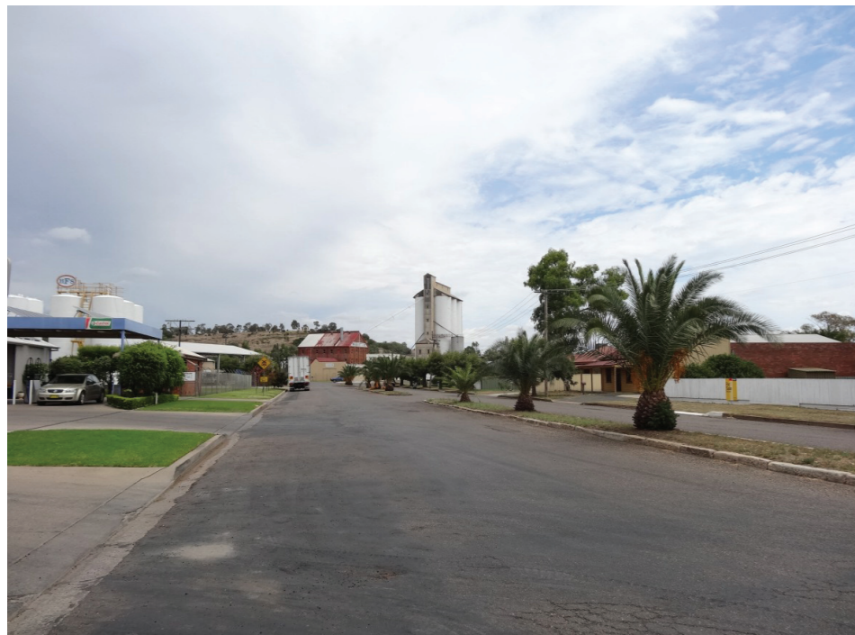
View looking east along Railway Avenue with the Mill in the background
