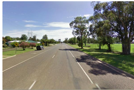
Figure 2.10: View Street (looking north)
