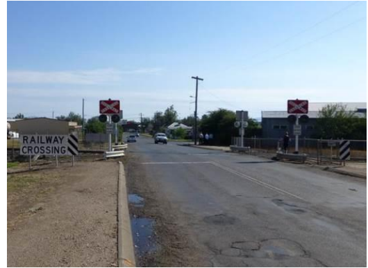
Figure 2.15: New Street at-grade crossing (looking north)
