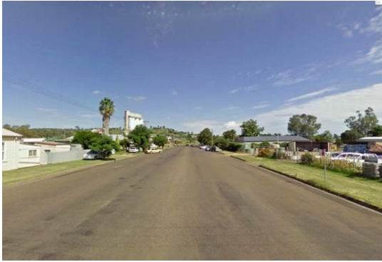
Figure 2.7: Barber Street (looking north-west)
