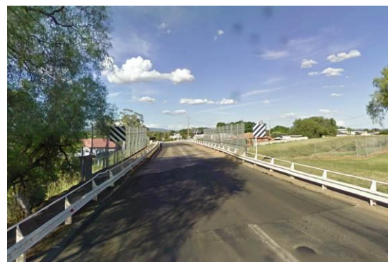
Figure 2.13: Abbott Street Bridge (looking northeast)
