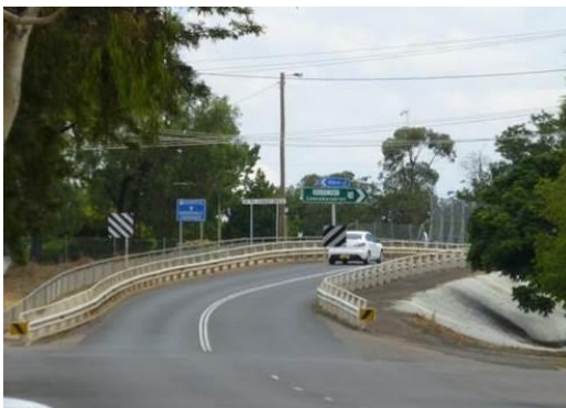
Figure 2.12: Abbott Street Bridge (looking southwest)
