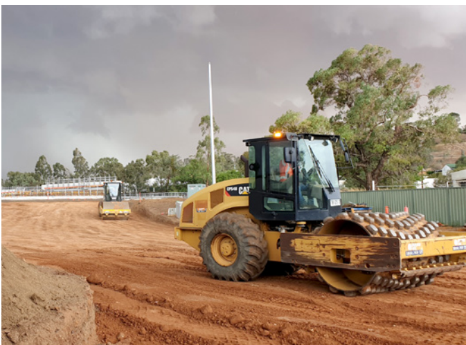
Earthworks to build the local road connection
