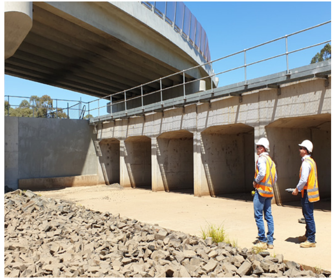
View of bridge and culverts
