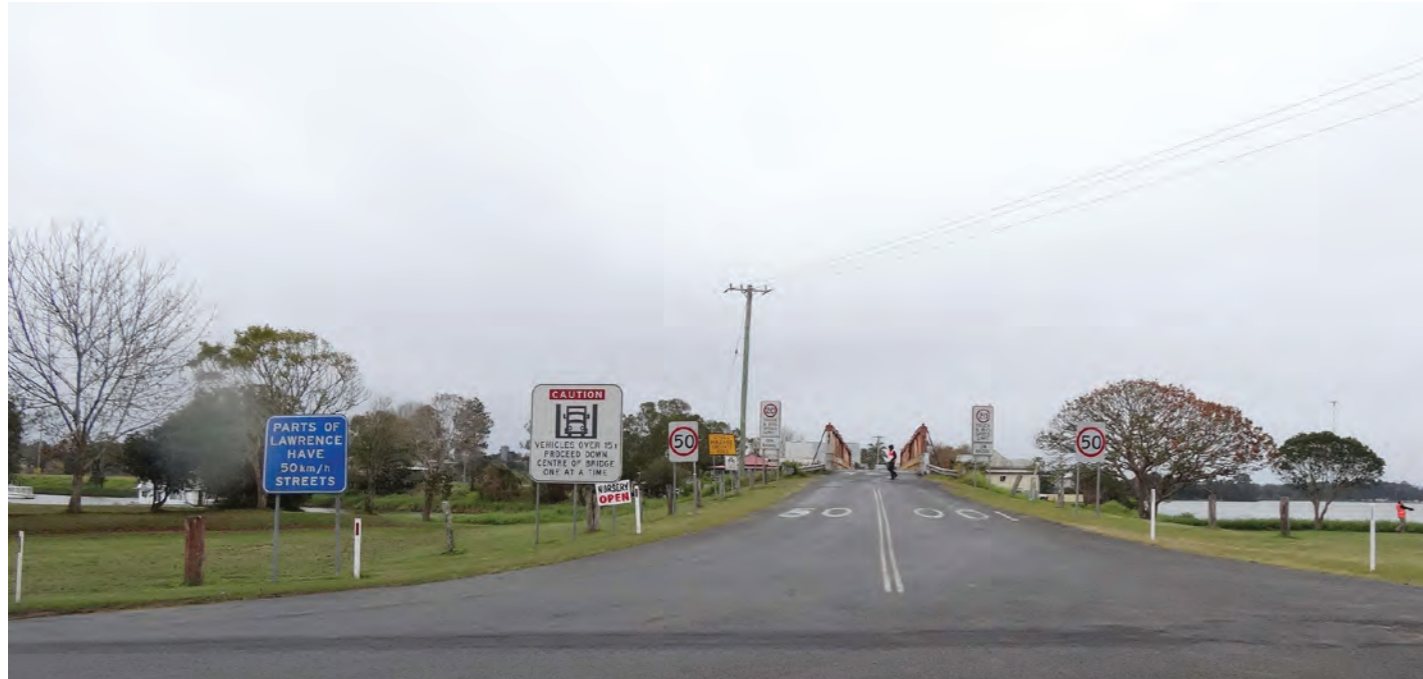
1 Approach to the existing Sportmans Creek bridge, with first glimpse of village from to right. Proliferation of safety signs.
