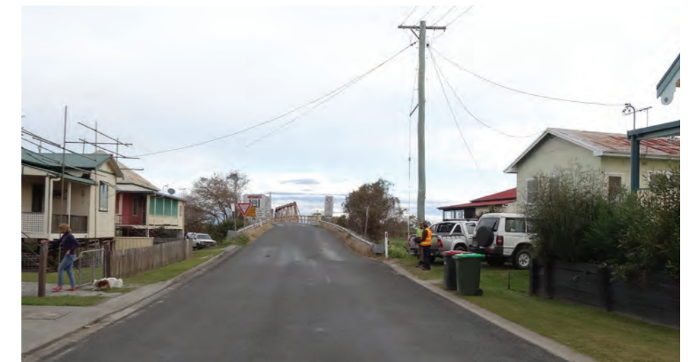
The bridge demolition provides opportunity for streetscape improvements to Bridge Street. The southern end of Bridge Street would benefit with some small scale street trees. The area closest to the old bridge offers potential for having narrowed pavement, and creation of a community meeting place- e.g. viewing deck with fishing potential and interpretation signage, with seating.
