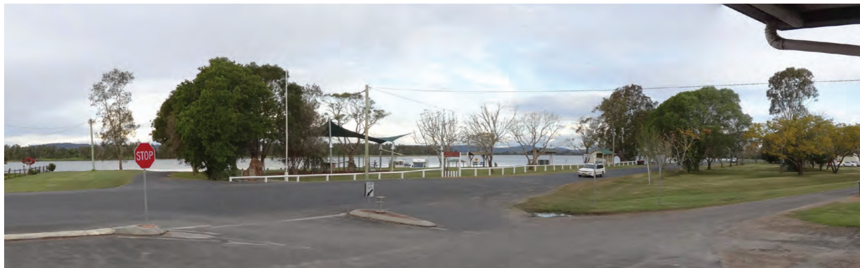
Framing this impressive view to the Clarence River from the northern town entry is important, as well as retaining the avenue trees to the right along Grafton Street.
