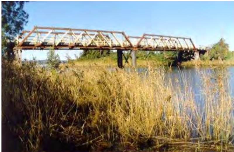
Sportsmans Creek Road bridge
