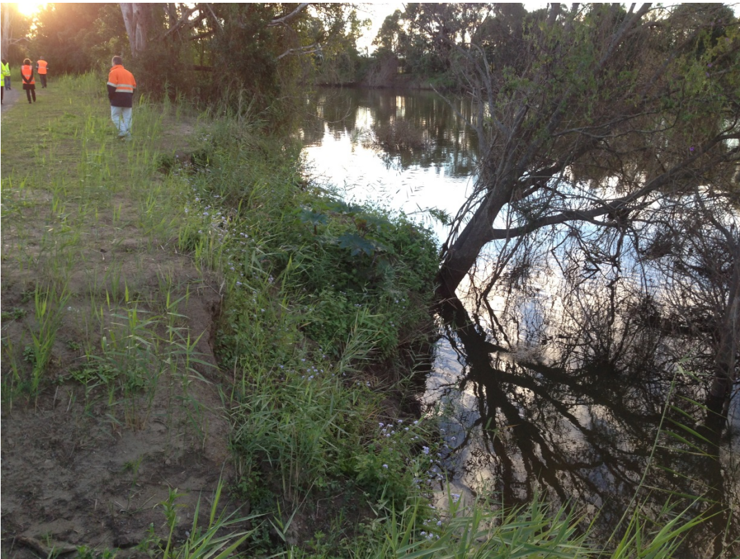
Photo 4: Upstream at existing bridge, looking north west showing recent river bank instability/erosion.
