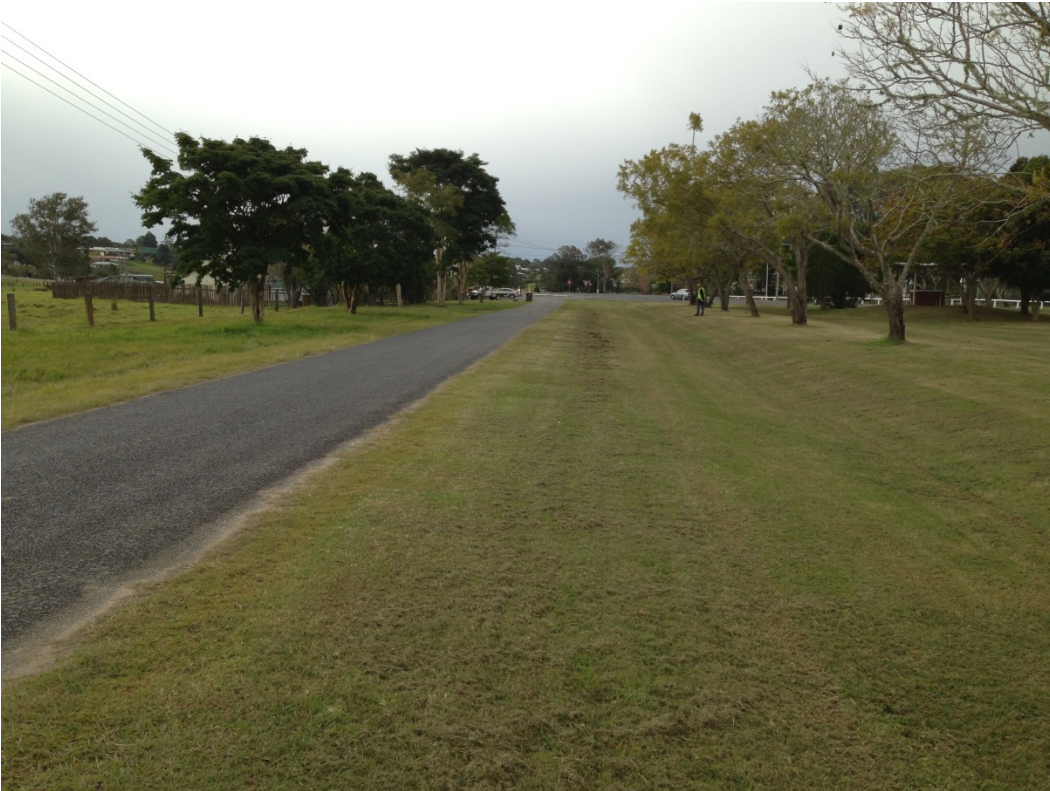
Photo 1: Looking north along Grafton Street showing light duty pavement construction.
