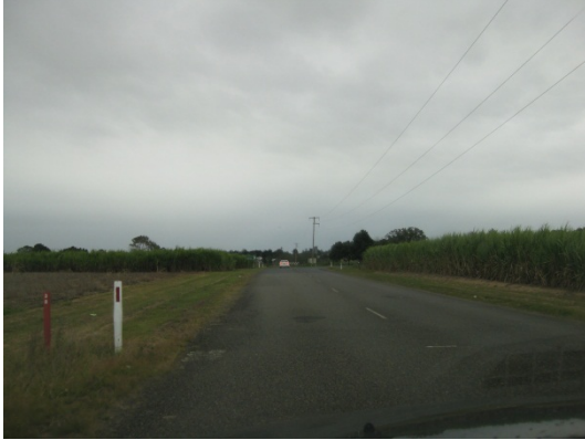
Figure 2.3: Grafton-Lawrence Road (looking north)
