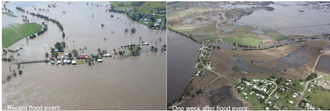
Figure 5.7 Recent flood event photos (Source: Roads and Maritime)
