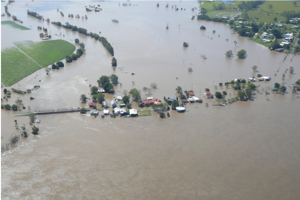
Figure 5.7 - Recent flood event (Source: Roads and Maritime)
