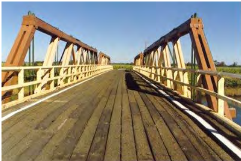
Sportsmans Creek Road bridge
