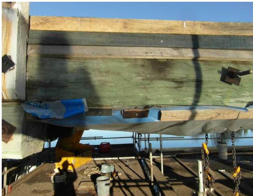
Plate 5.4 McFarlane Bridge microbat exclusion viewed from side-on
