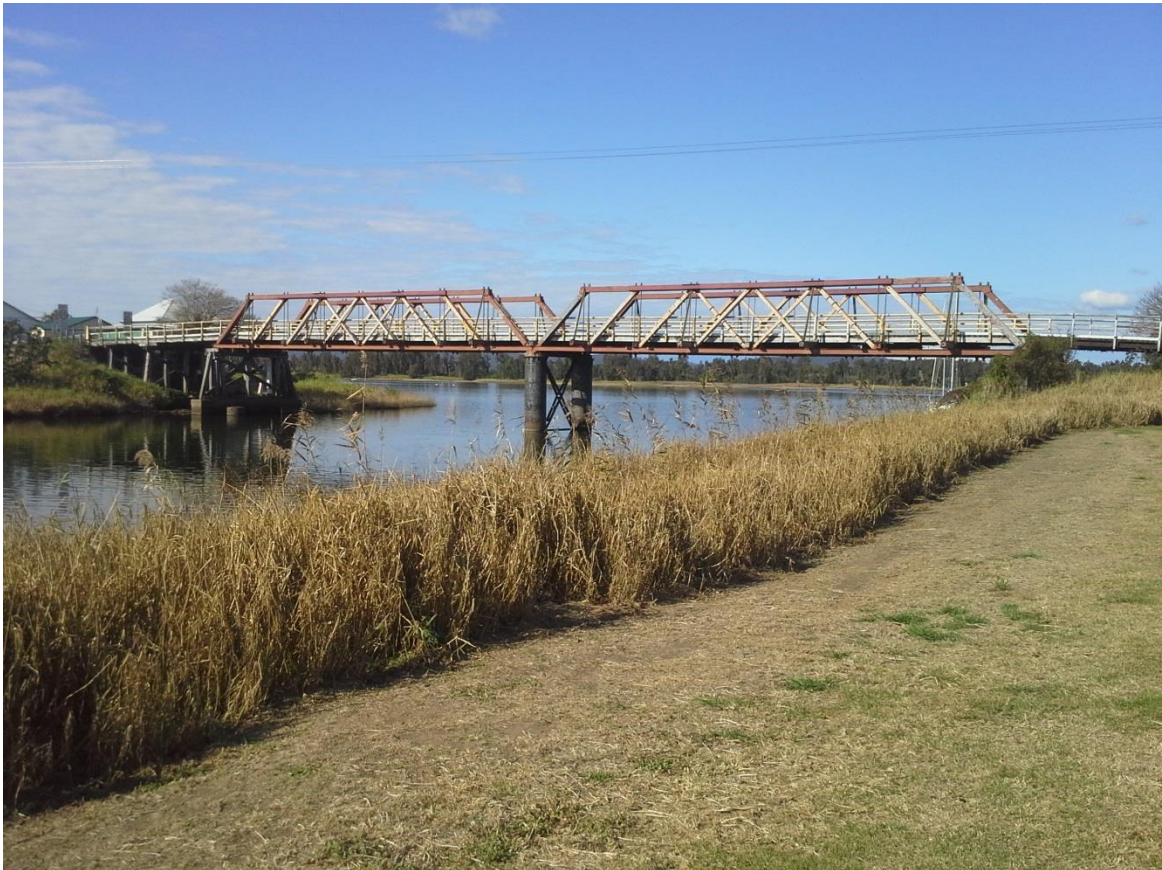
Figure 3-4 Photograph of existing bridge on Sportsmans Creek
