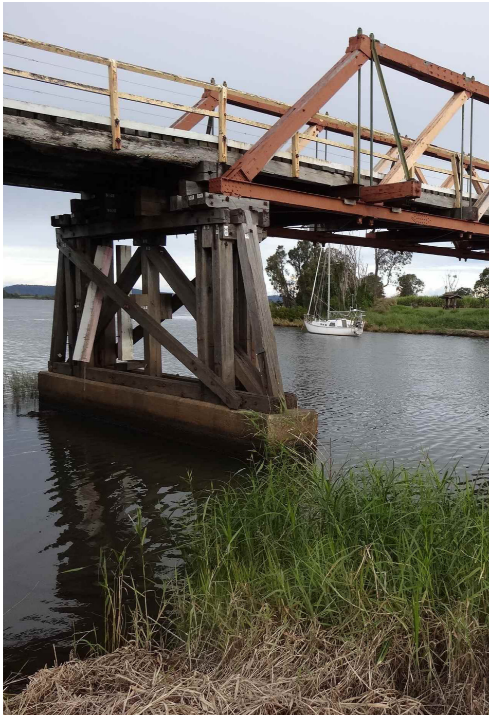
Figure 1.46 Contextual View - Sportsmans Creek bridge
