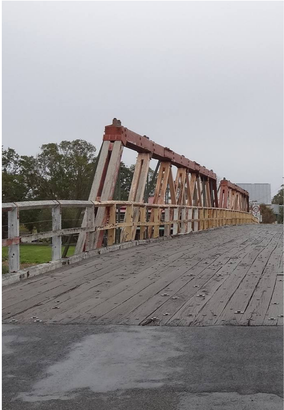
Figure 1.48 Contextual View - Sportsmans Creek bridge
