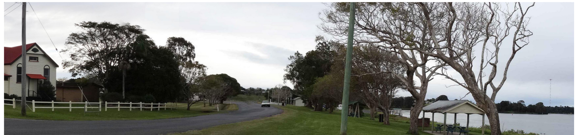
Figure 1.45 The Heritage Village has special built form, landscape and contextual character that must be respected. View corridors to water between housing and across parklands are special elements through the town.
