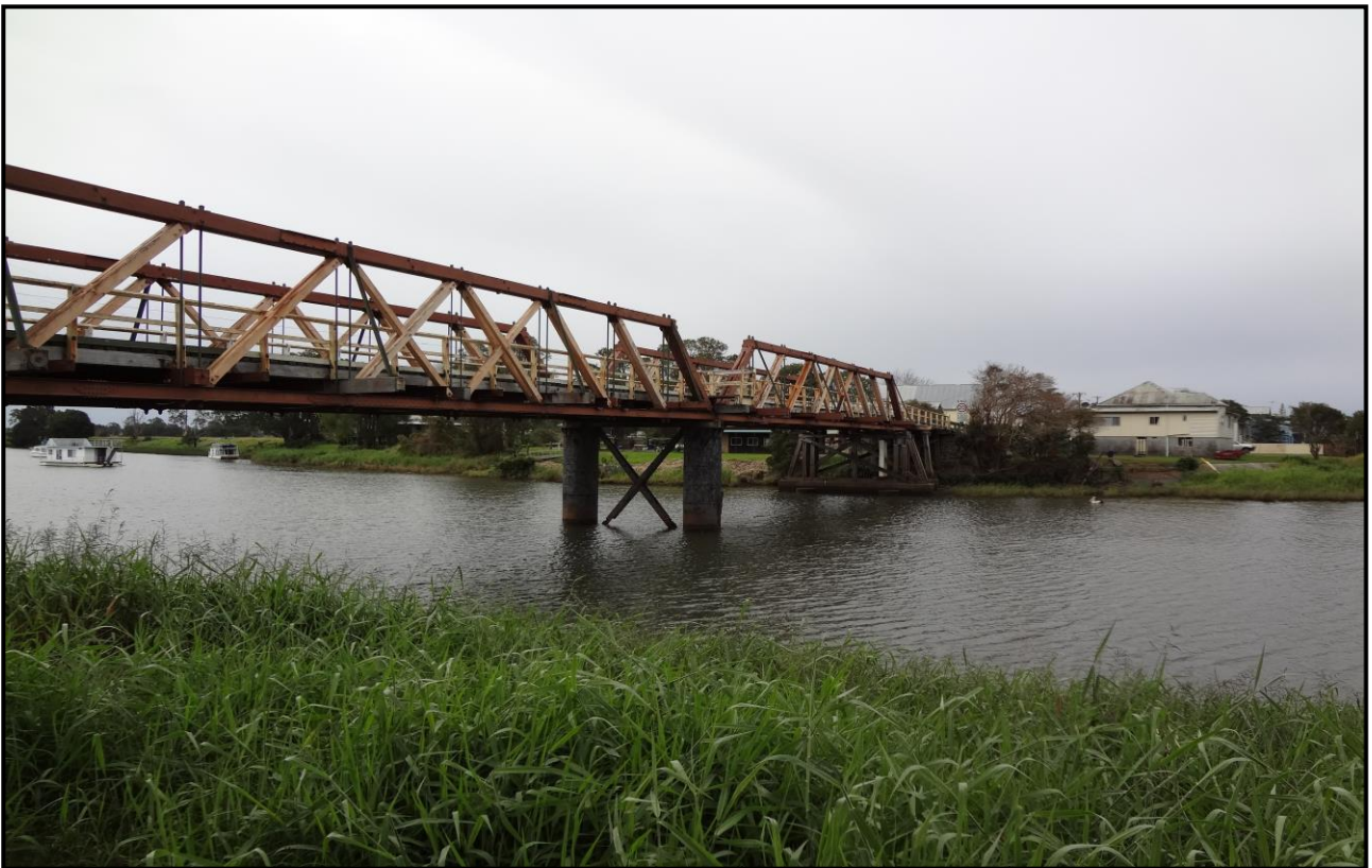
Plate 3.2: Sportsmans Creek Bridge looking towards the northern abutment
