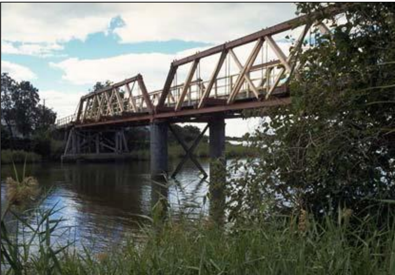
Plate 6.13: Sportsmans Creek Bridge in May 1996 (Source: Department of the Environment)
