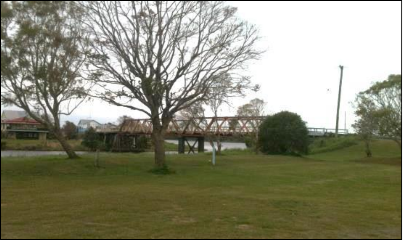
Plate 6.1: View north-east towards Sportsmans Creek Bridge showing isolated trees within Flo Clark Park
