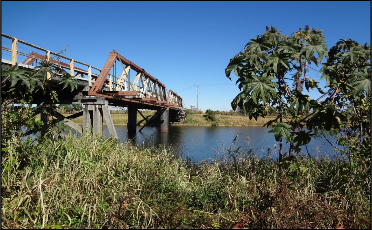
Plate 3.3: Sportsmans Creek Bridge looking towards the southern abutment
