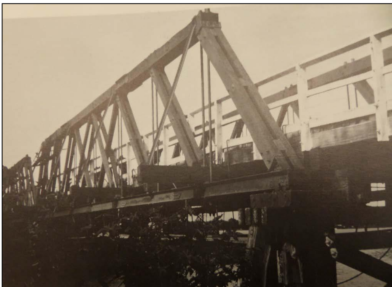
Plate 6.11: Dare truss bridge at Sportsmans Creek, 1911 (undated image) Source: Colin O'Connor Spanning Two Centuries, historic bridges of Australia , Queensland University Press, 1985)
