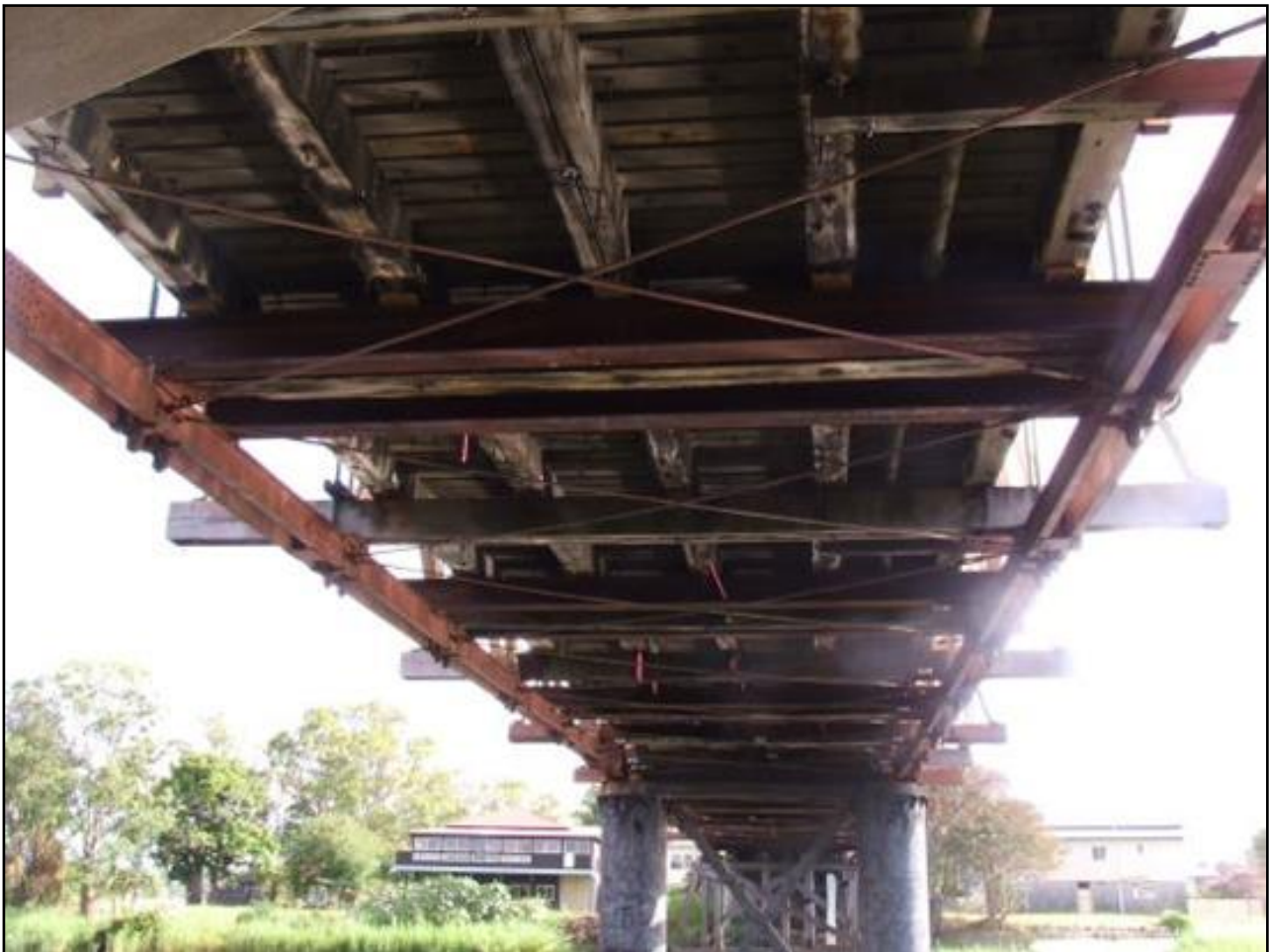
Plate 6.5: View north showing underside of Sportsmans Creek Bridge
