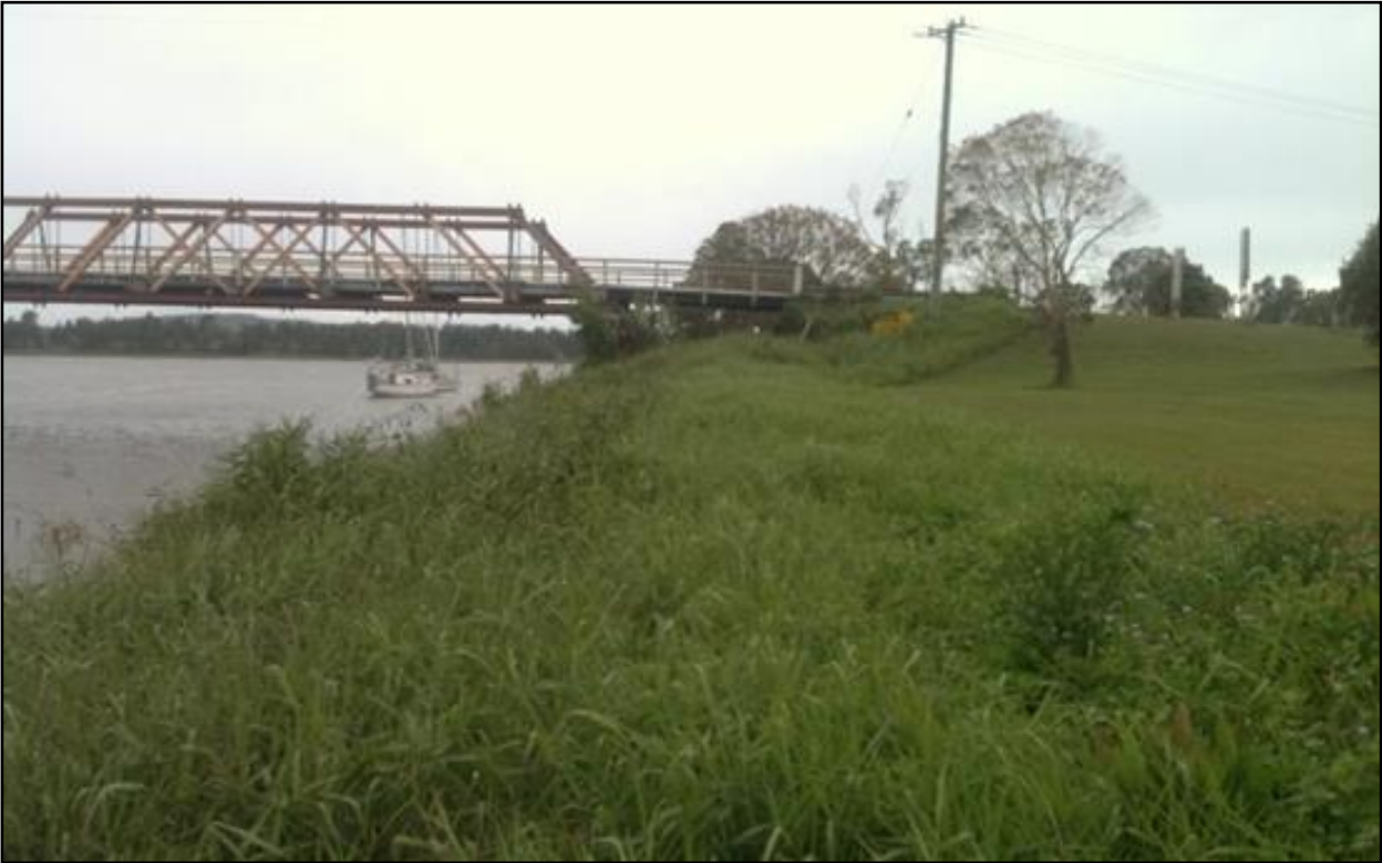
Plate 6.3: View east showing un-mown riparian vegetation
