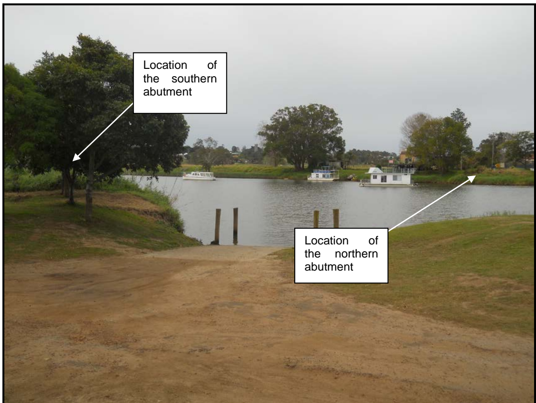
Plate 3.2 Looking at the southern abutment across Sportsmans Creek from Flo Clark Park
