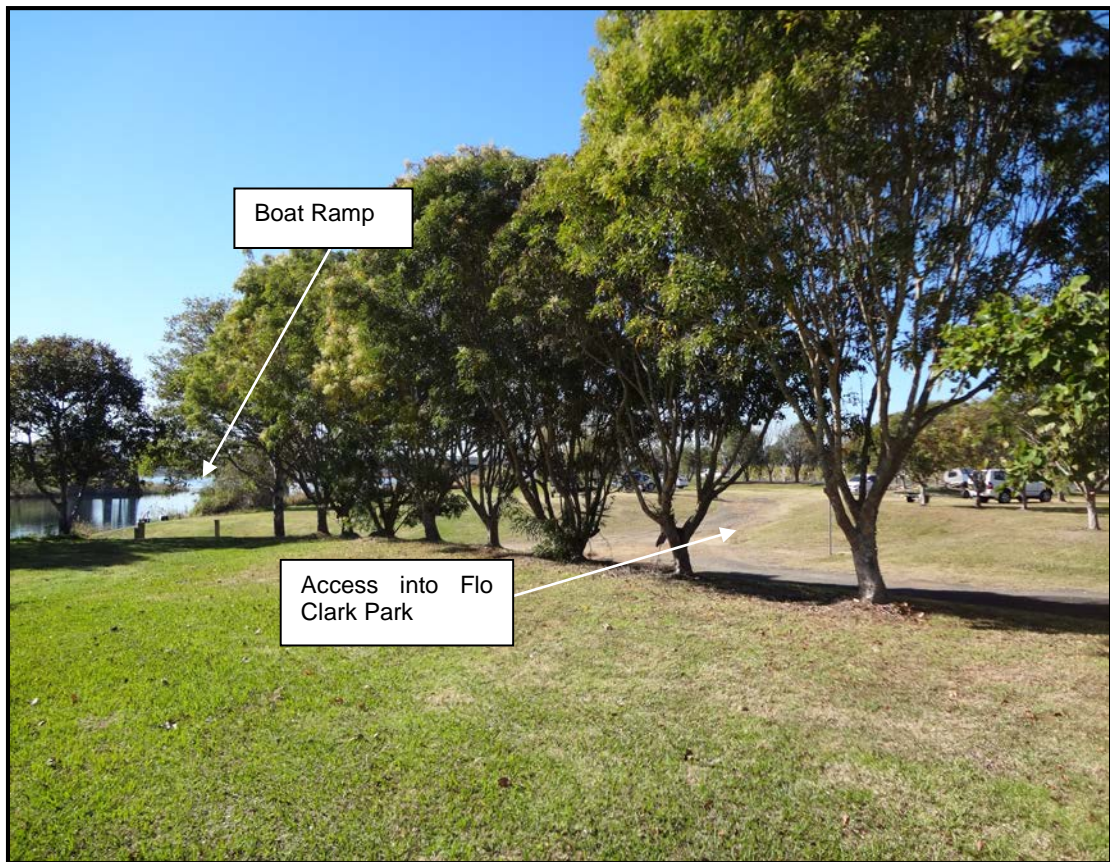
Plate 3.14 Existing access into Flo Clark Park and Boat Ramp
