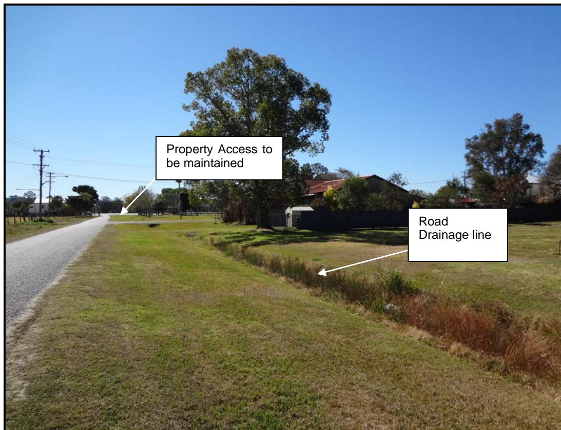
Plate 3.7 Drainage and property access to be upgraded on Grafton Street
