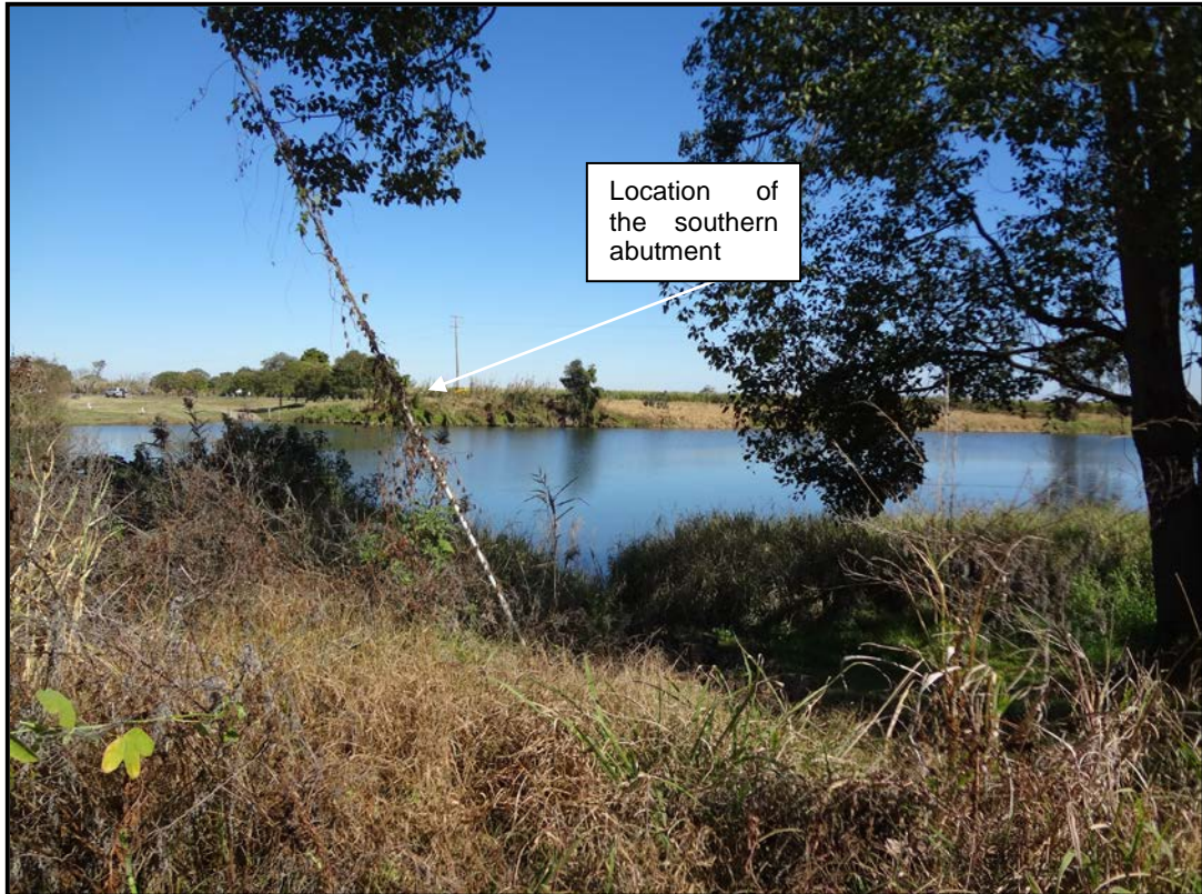
Plate 3.3 Standing on the location of the northern abutment, looking towards the south over Sportmans Creek along the alignment
