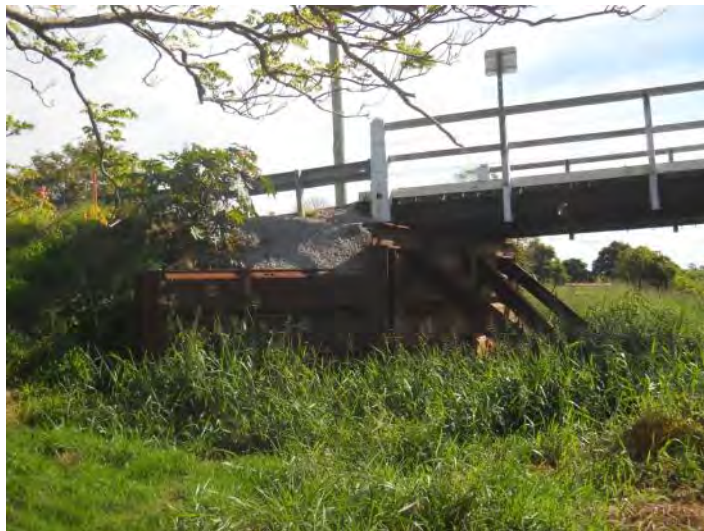
Plate 2.6 Southern abutment to be removed
