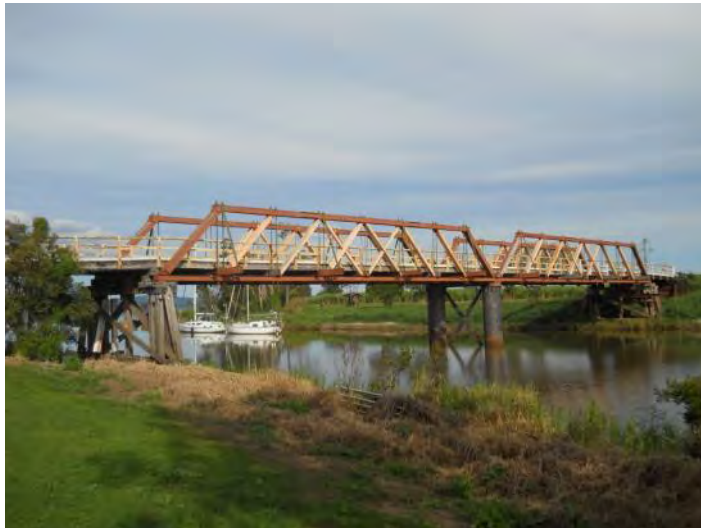
Plate 2.1 View north-west toward Sportsmans Creek Bridge from Sportsmans Park
