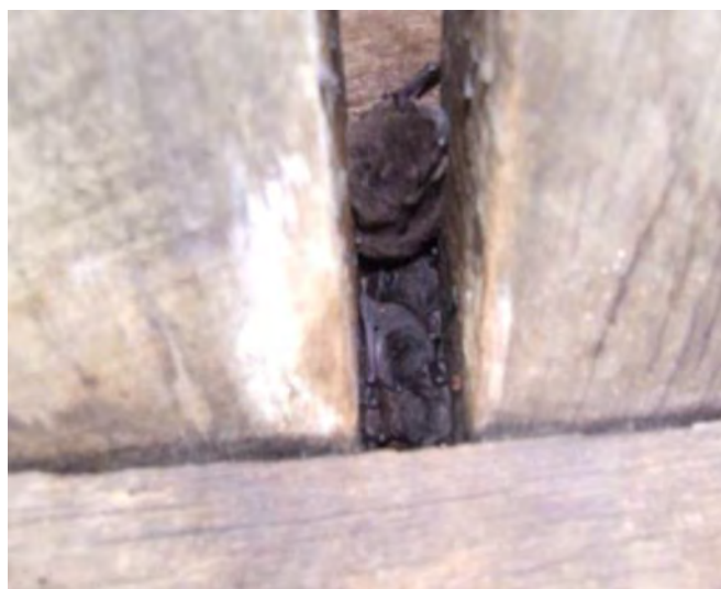
Plate 4.3 Large-footed Myotis in bridge decking
