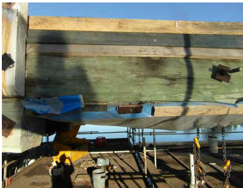
Plate 2.2 McFarlane Bridge microbat exclusion viewed from side-on
