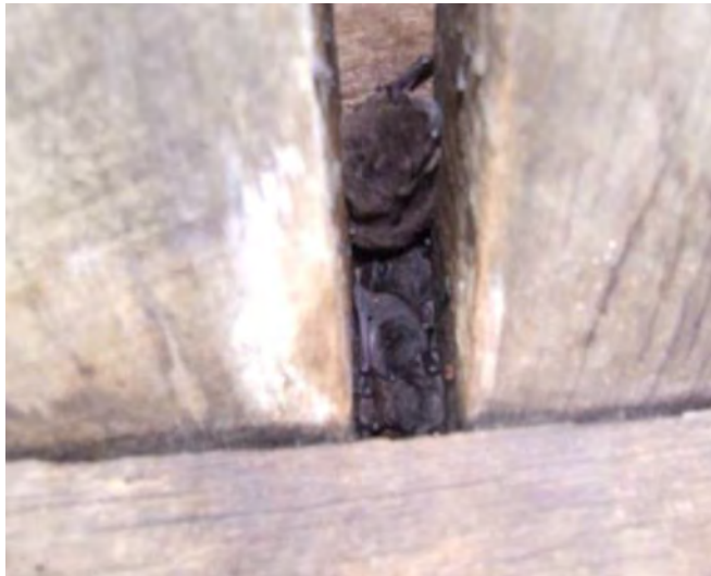
Plate 3.7 Large-footed Myotis in bridge decking
