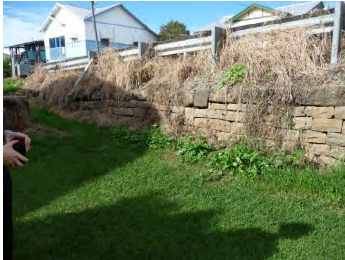
Plate 2.5 Northern abutment to remain insitu
