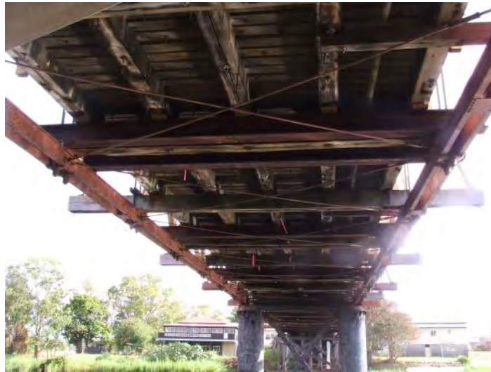
Plate 3.5 View north showing underside of Sportsmans Creek Bridge
