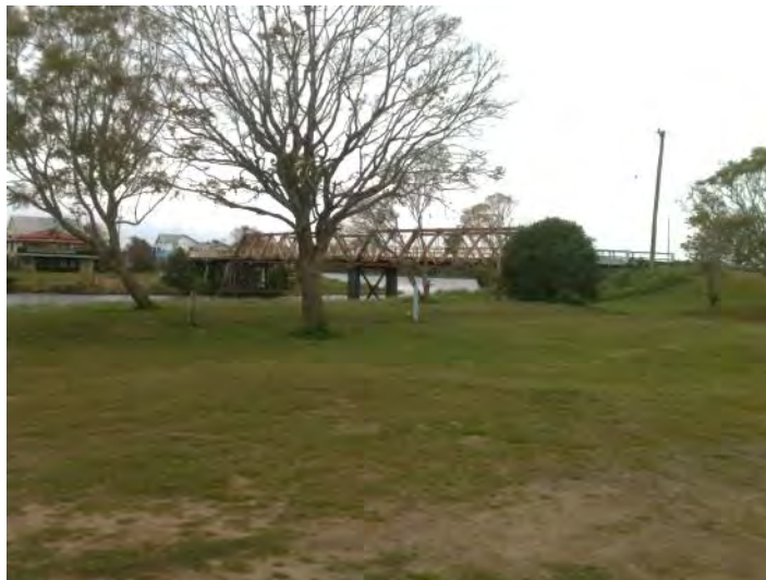
Plate 3.1 View north-east towards Sportsmans Creek Bridge showing isolated trees within Flo Clark Park
