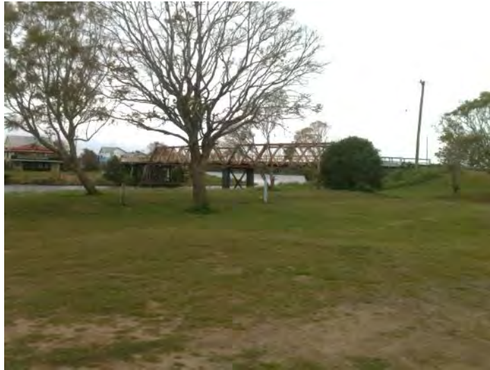
Plate 2.7 View north-east towards Sportsmans Creek Bridge showing isolated trees within Flo Clark Park
