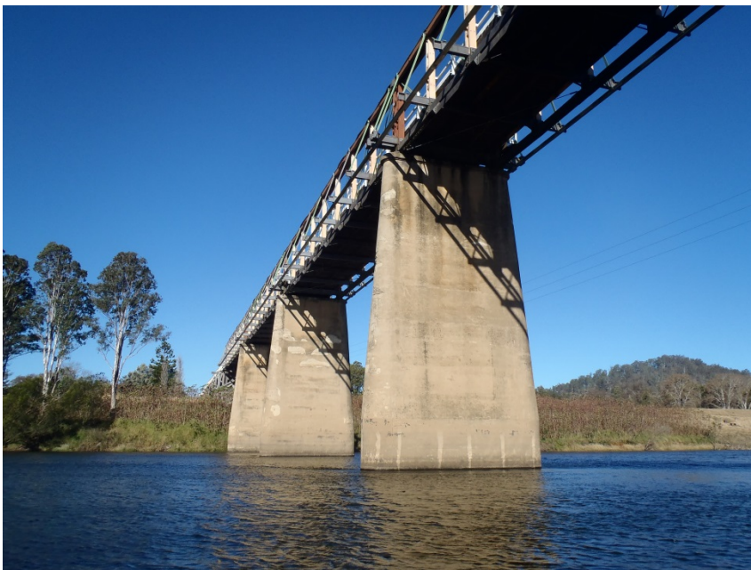
Figure 3: Existing bridge (view towards eastern bank)
