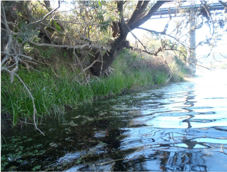
Figure 9: Riparian vegetation and bank structure on western bank of new bridge alignment
