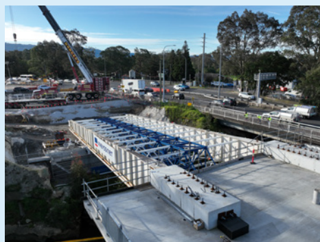
Left: The launch nose about to be dismantled having reached the northern foreshore. Right: Sunrise view of the bridge and the rock platform from the casting yard.
