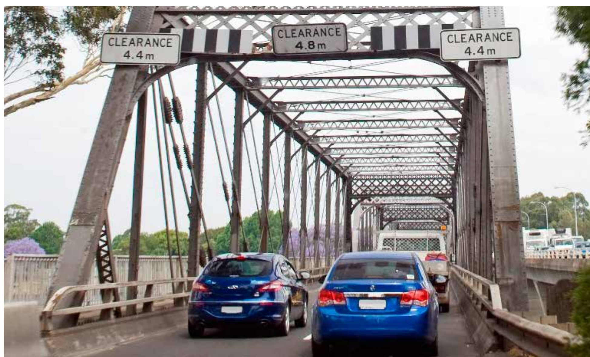
The old Nowra Bridge looking south
