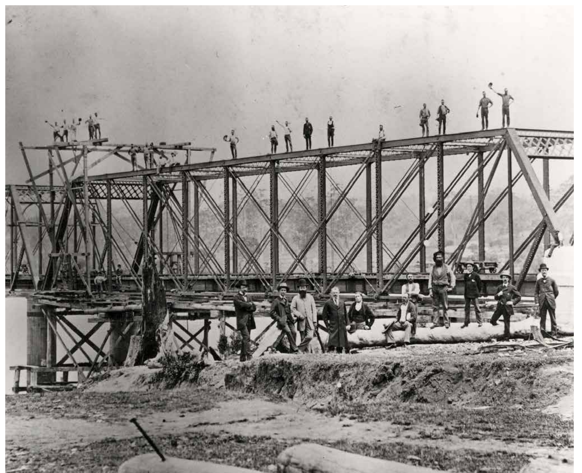
The old Nowra Bridge during its construction, around 1880.
