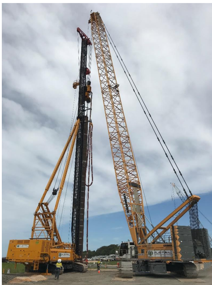
Photograph of piling rig on left and crane on right
