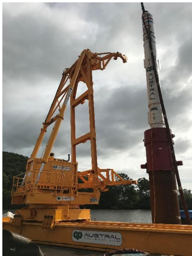
Photograph of piling hammer
