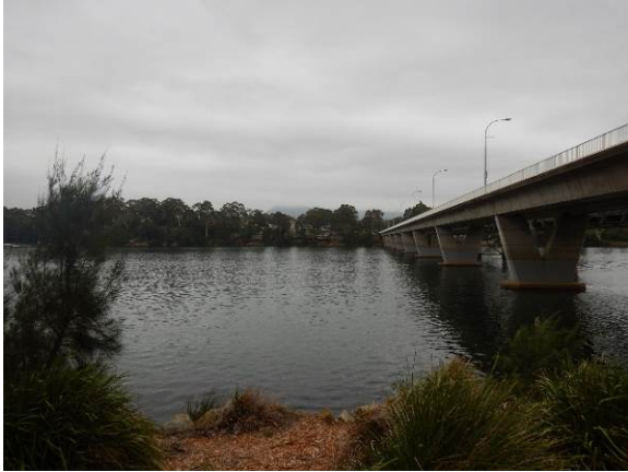
Figure 4.11: View north across the Shoalhaven River from the approximate location of the proposed new bridge, next to the northbound concrete bridge (seen right)
