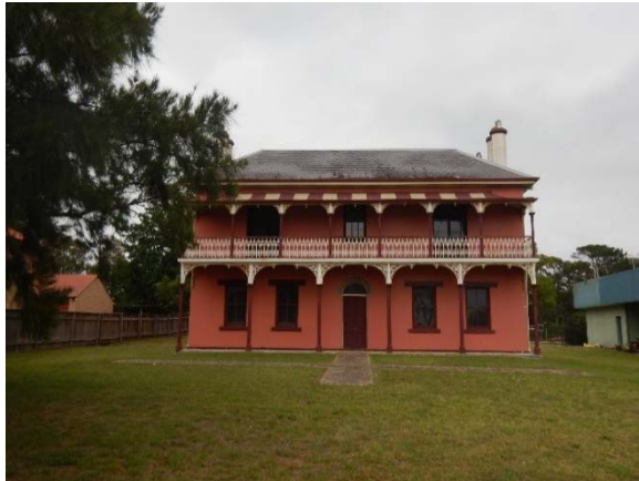
Figure 5.1: View of east (main) façade of Graham Lodge
