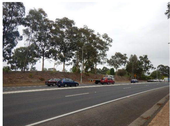
Figure 4.22: View north west across Princes Highway to approximate site of proposed intersection upgrade at Bridge Road
