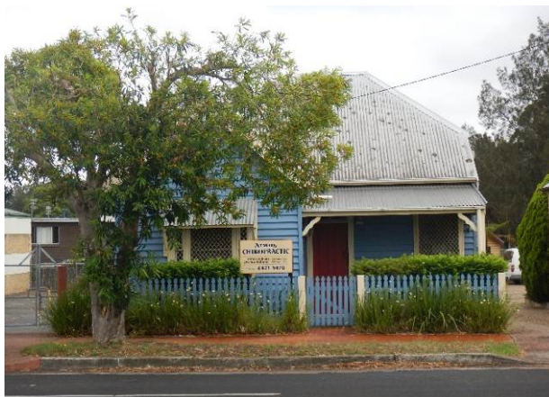
Figure 5.12: View to 'Late Victorian weatherboard residence' from southern side of Moss Street
