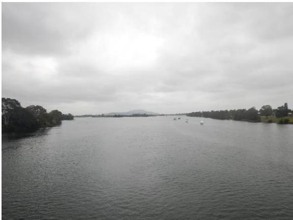
Figure 4.9: View east across the Shoalhaven River from the pedestrian walkway attached to the Nowra truss bridge
