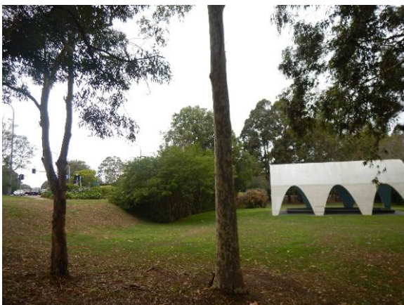
Figure 4.15: View south alongside Princes Highway at the approximate location of the proposed southern approach to a new Nowra bridge, Captain Cook Memorial seen to right
