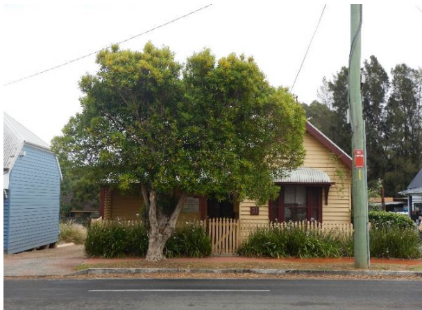
Figure 5.13: View to ‘Late Victorian weatherboard cottage’ from southern side of Moss Street
