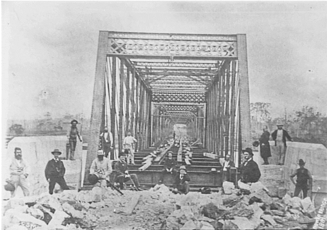
Figure 3.6: Workers at the approach to the Nowra Bridge, 1881. Source: Wollongong City Library
