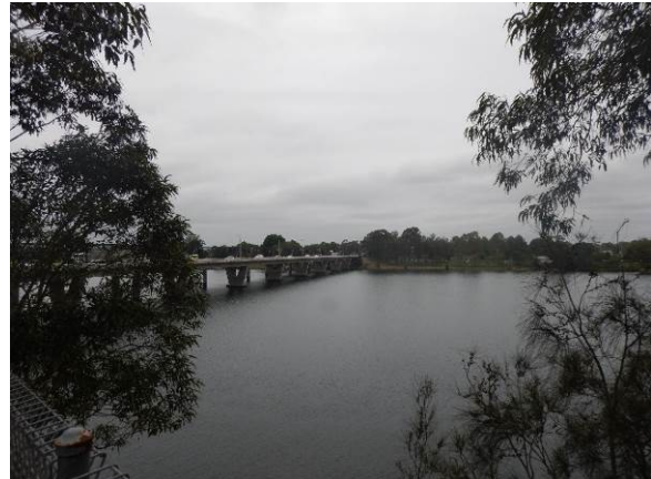
Figure 4.2: View south east across the Shoalhaven River to Nowra Bridge, showing approximate site of proposed bridge
