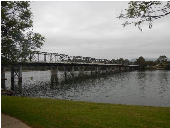
Figure 5.2: View of north west of the truss bridge
