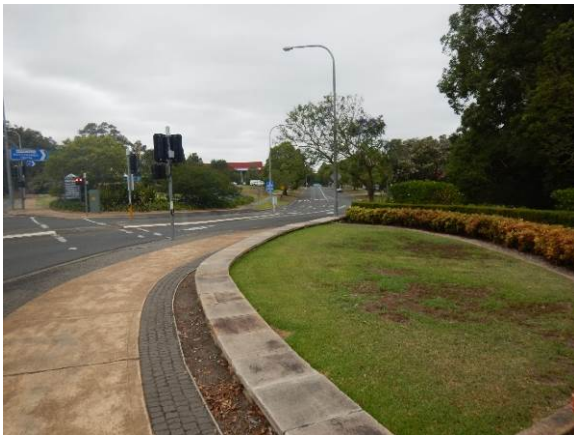
Figure 4.19: View south west at intersection of Princes Highway with Bridge Road, approximately location of proposed southern approach to a new Nowra bridge
