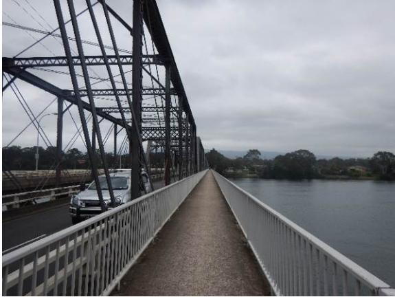
Figure 4.5: View north along the pedestrian walkway off the Nowra truss bridge (seen left)
