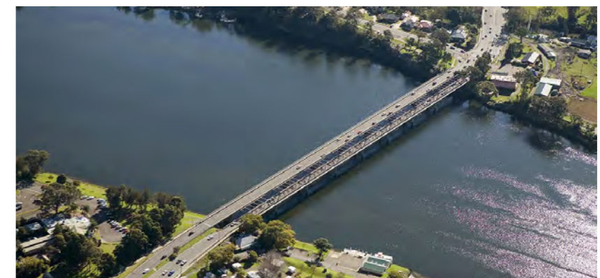
Figure 23. Aerial view of the Shoalhaven River and the existing southbound and northbound bridges looking northwest
