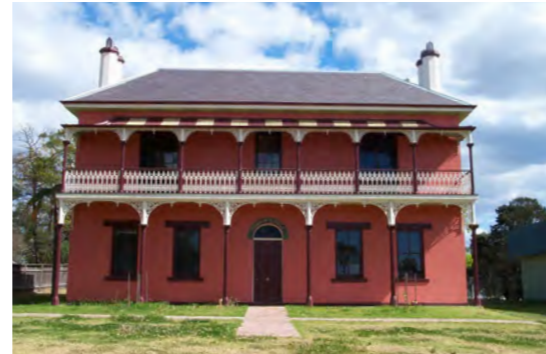
Figure 24. Graham Lodge Source: www.shoalhaven.nsw.gov.au
