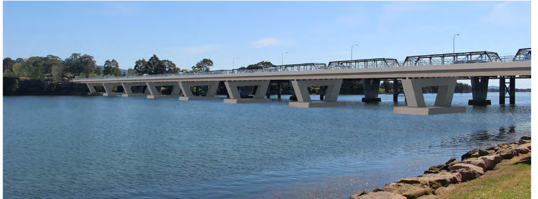
Figure 83. Viewpoint 6 looking north-east from the southern foreshore towards Nowra Bridge - Proposed (Option 2)
