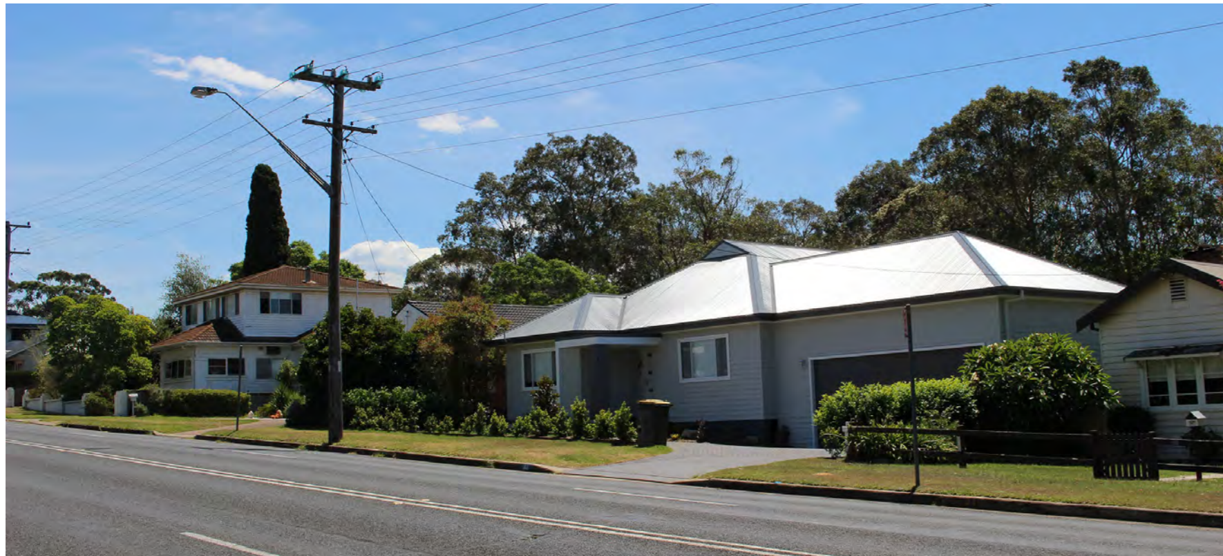
Figure 68. Typical residential dwellings on Illaroo Road
