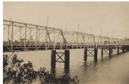
Figure 25. Existing heritage truss bridge Source: http://scourbrittfamily.files.wordpress.com/201302nowra
