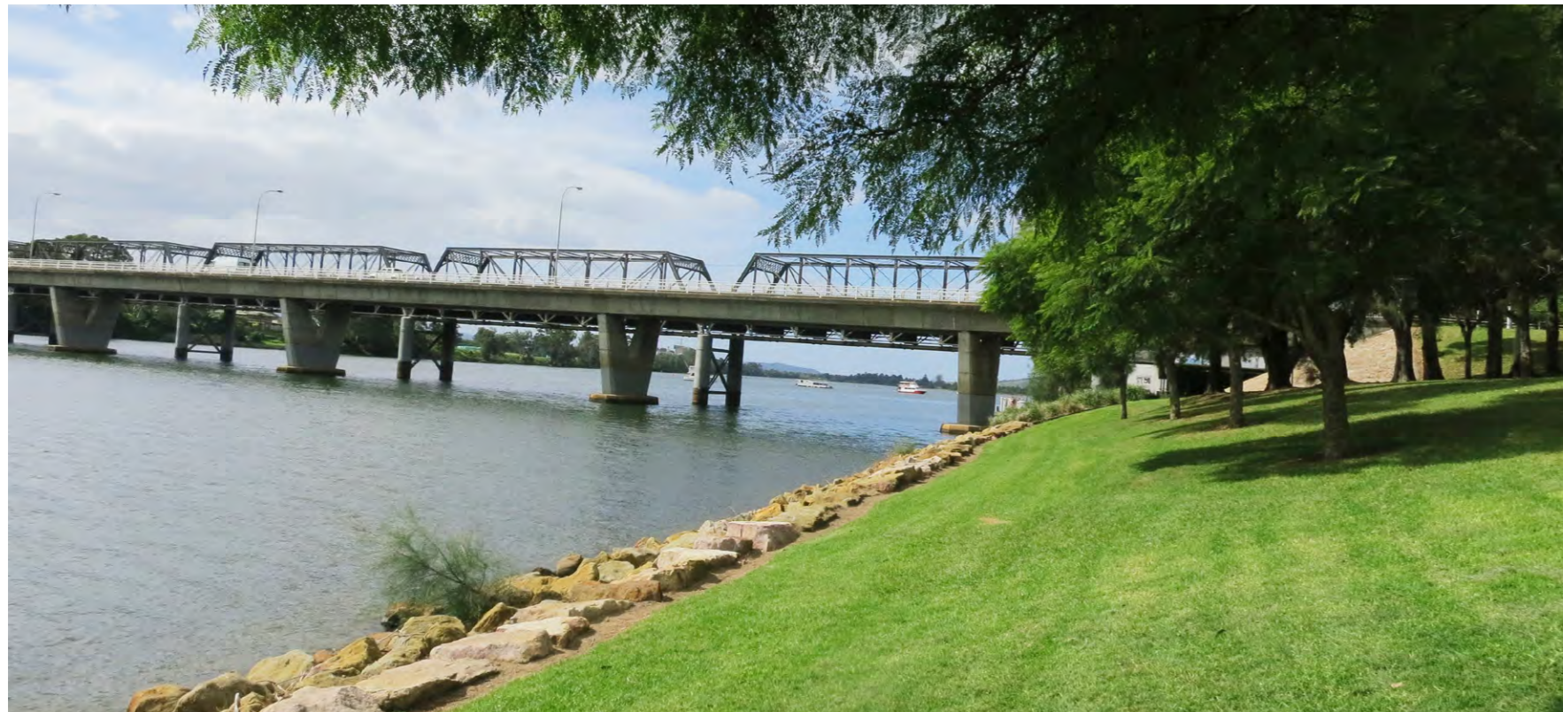
Figure 70. Foreshore open space looking east towards the existing bridge structures
