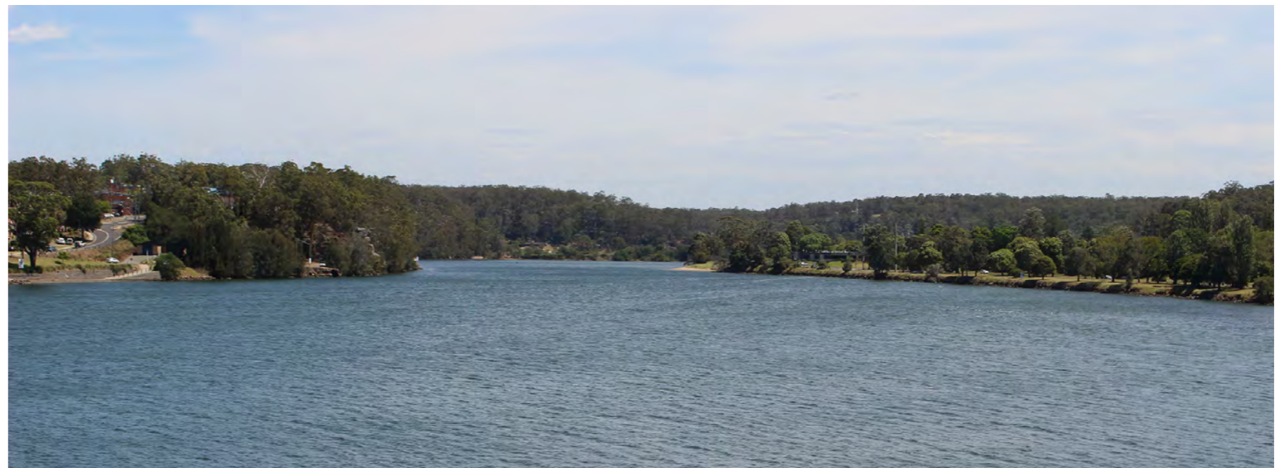
Figure 29. View from the existing northbound bridge looking west
