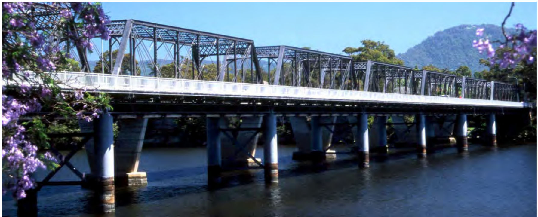
Figure 8. Existing southbound bridge - Heritage truss structure Source: https://c1.staticflickr.com/5/4040/4621053538_910bc5ddec_b.jpg
