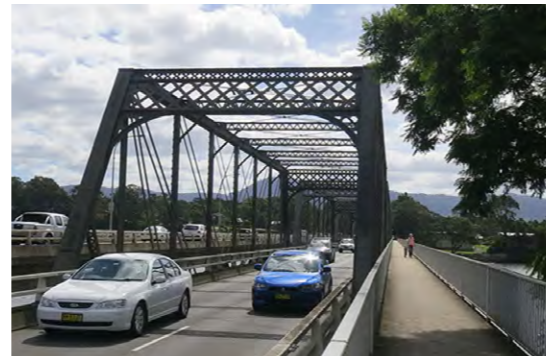
Figure 15. Shared path attached to heritage truss bridge
