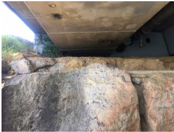
Photo 7: Lattice style retaining wall supporting fill material along the road corridor
