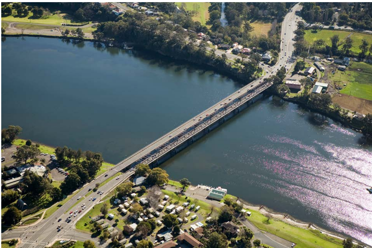
Figure 1-1 Princes Highway crossings of the Shoalhaven River (looking north west)
