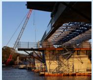
Launch nose being launched onto the bridge pier
