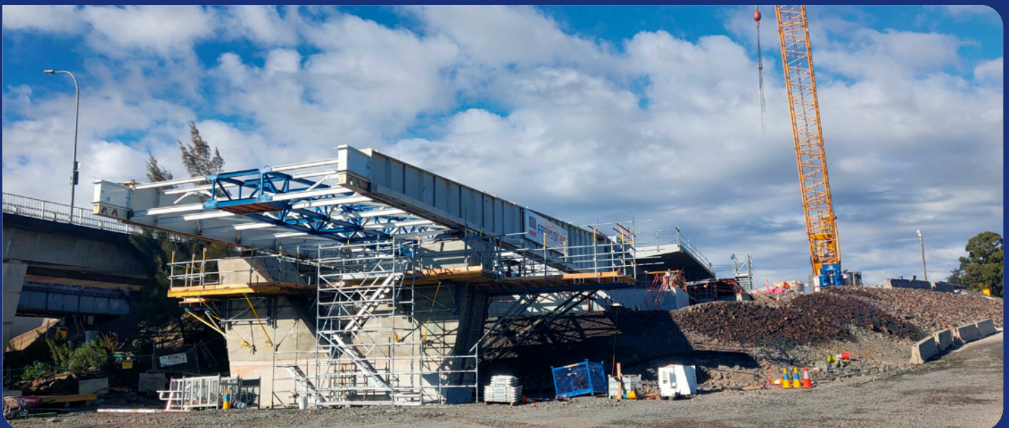
Launch nose being launched onto the bridge pier
