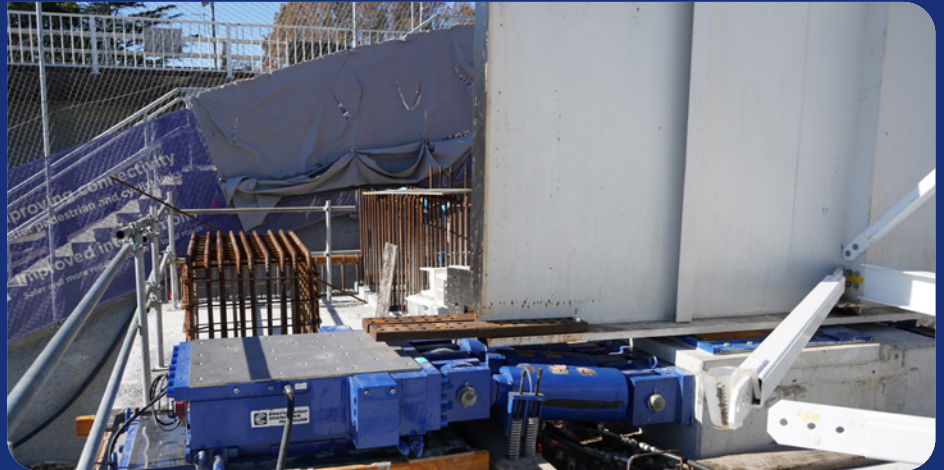
Hydraulic jack used to push the bridge into place
