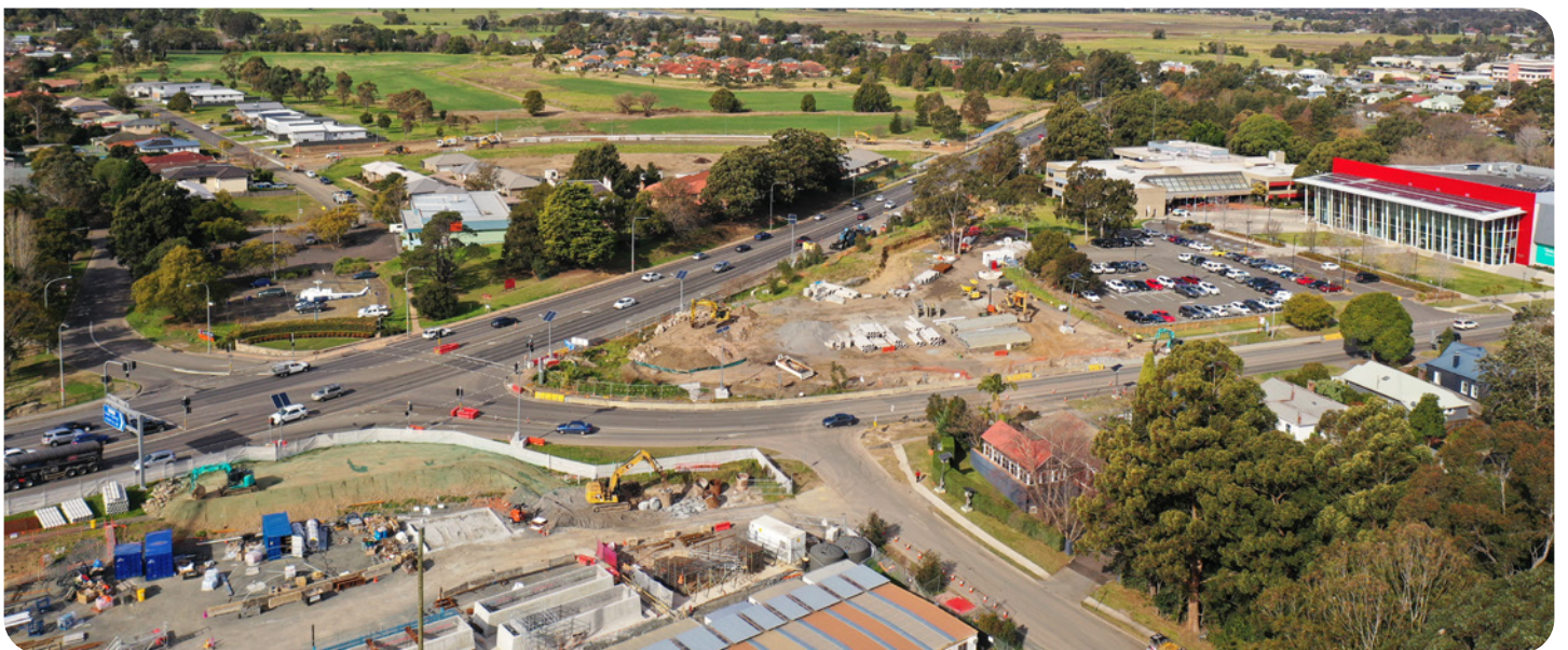
Intersection of Bridge Road and Princes Highway, looking east
