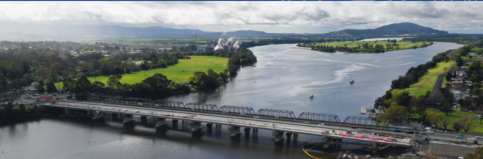
Aerial view of the Nowra Bridge project, looking east.
