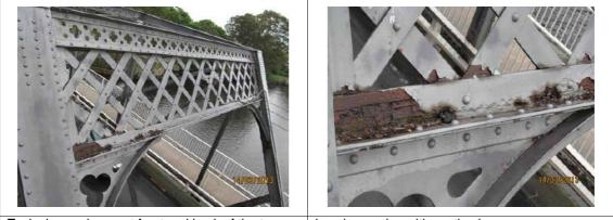
Typical cross brace at front and back of the truss. Local corrosion with section loss.
