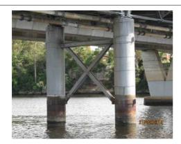
Pier 3 showing a missing bottom brace. The replacement of the missing brace is recommended as it helps to improve stability.
