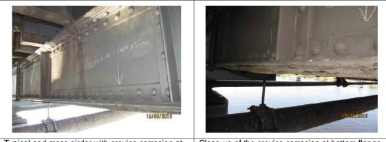
Typical end cross girder with crevice corrosion at bottom flange. Close-up of the crevice corrosion at bottom flange.
