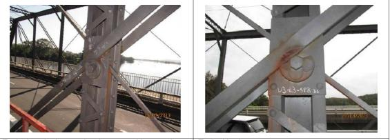
Typical vertical truss showing seat with corrosion Typical broken seat.
