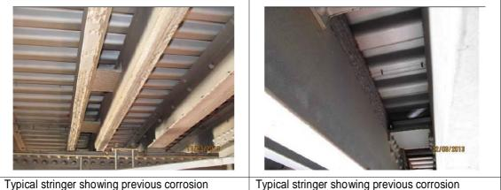
I ypical stringer showing previous corrosionI ypical stringer showing previous cdamage which had been repainted.damage inside stringer.
