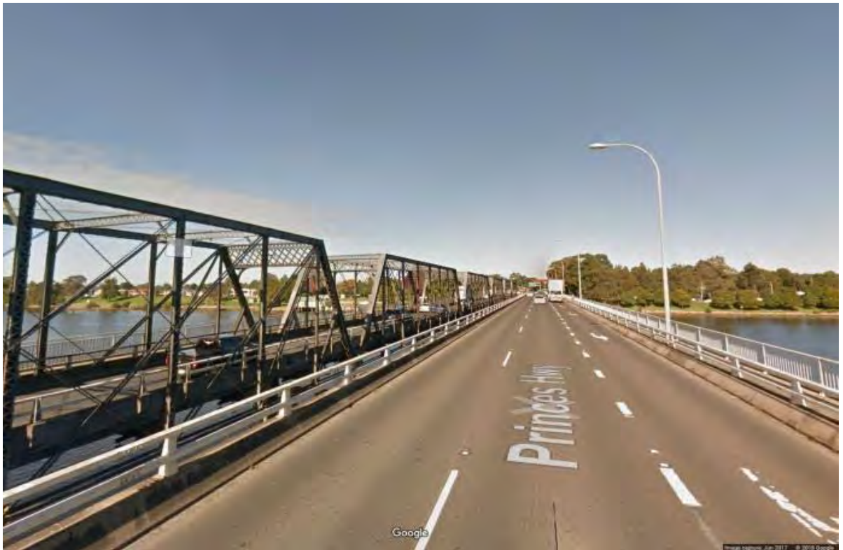
Figure 2-1: Existing Nowra Bridges (Source: Google Street View)
