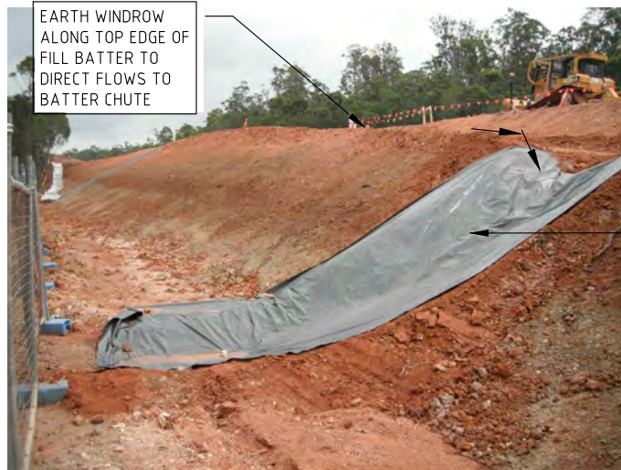
PHOTO 4 - EXAMPLE OF BATTER CHUTE
