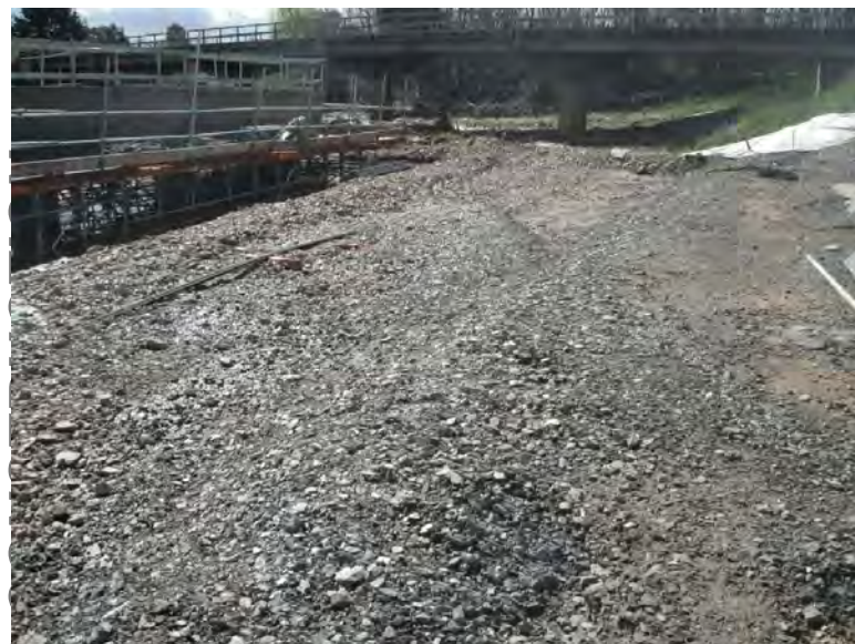
PHOTO 6 - EXAMPLE OF A PILING PLATFORM STABILISED SURFACE
