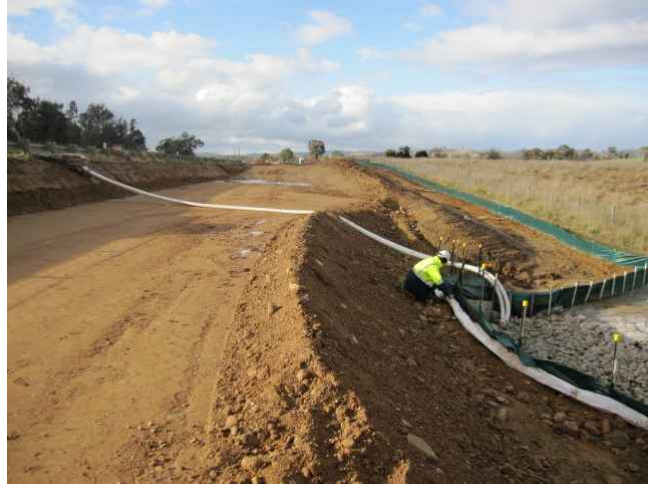
PHOTO 1 - EXAMPLE OF TEMPORARY PIPED CLEAN WATER DIVERSION INSTALLED PRIOR TO RAINFALL
