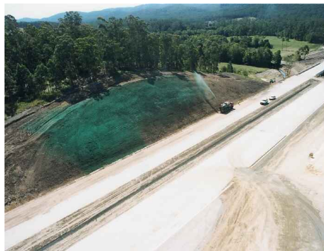
PHOTO 5 - TEMPORARY STABILISATION OF BATTERS WITH POLYMER
