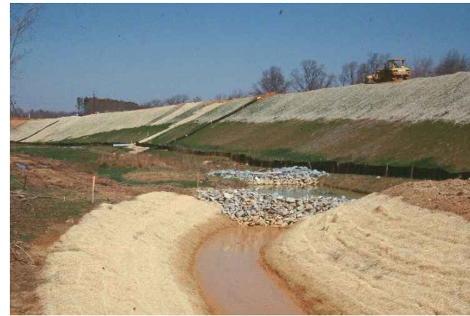
PHOTO 2 - PROGRESSIVE STABILISATION OF BATTERS AS WORKS PROGRESS
