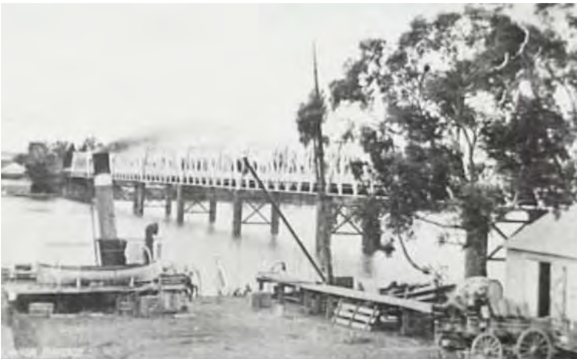
Plate 4.3 Bomaderry Wharf, undated (Wollongong Library)
