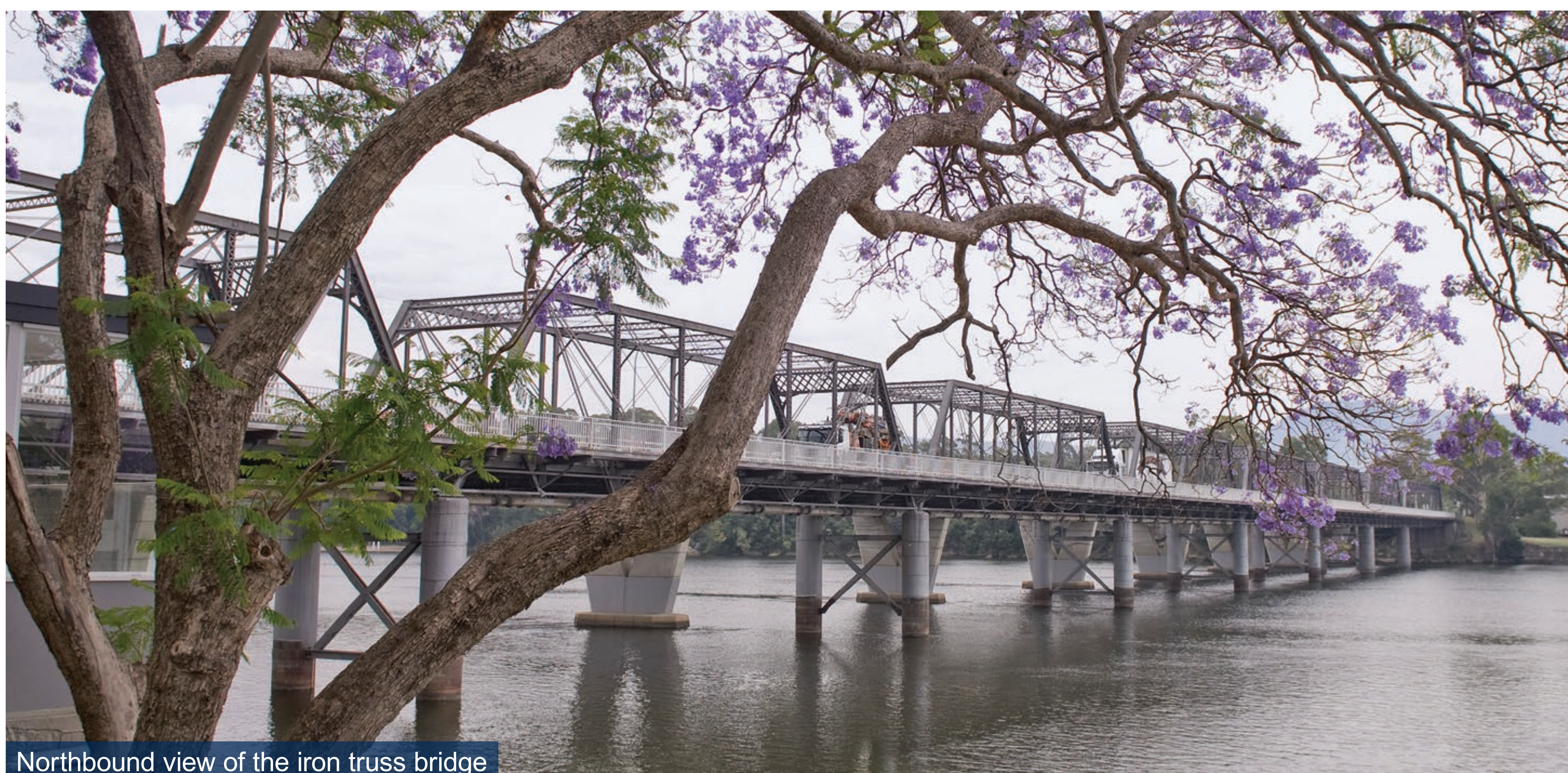
Northbound view of the iron truss bridge
