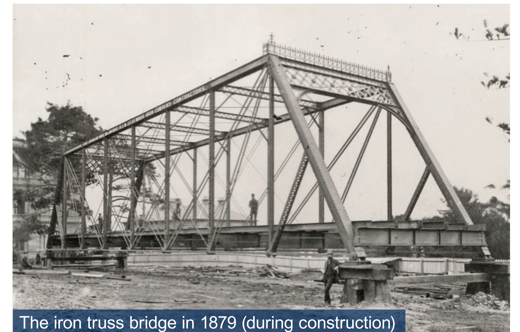
The iron truss bridge in 1879 (during construction)
