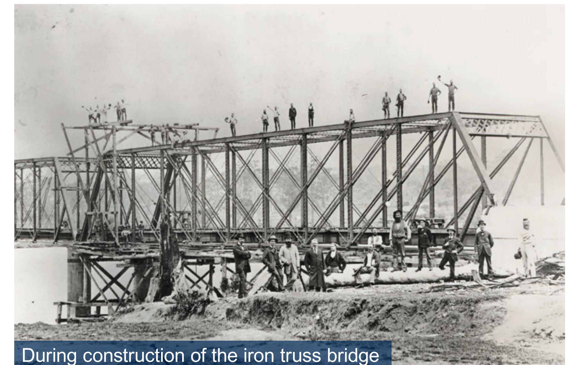
During construction of the iron truss bridge
