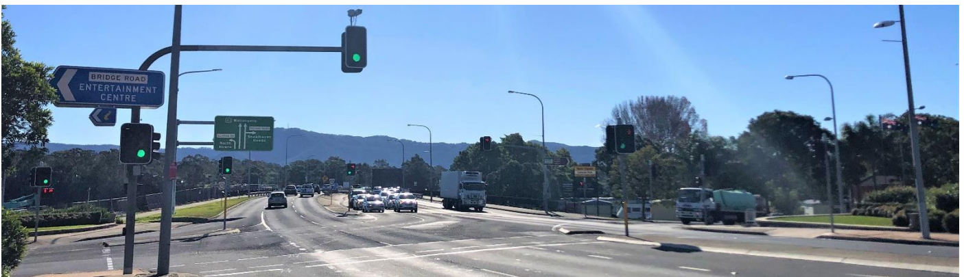
Night work will occur on the Princes Highway, Nowra
