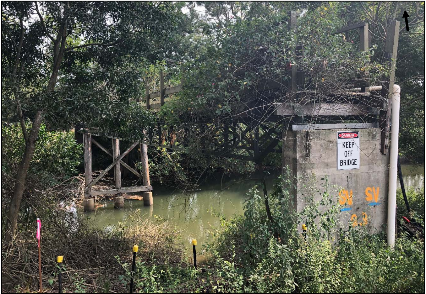
Figure 3-6 Looking north to the Bomaderry Creek footbridge (Source: Roads and Maritime, 2019).
