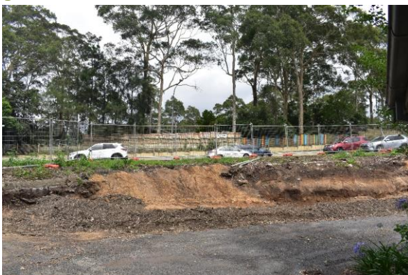
Figure 31. View west towards area of works from driveway.
