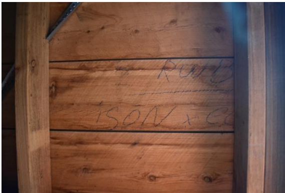
Figure 27. View of interior and carpenters' mark of c.1990s shed.
