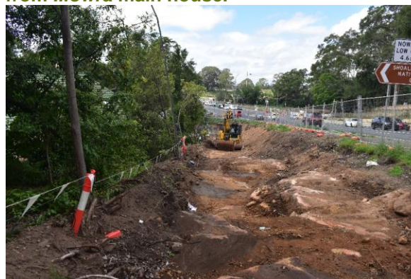
Figure 32. View south towards area of bulk excavation.
