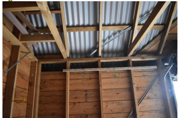
Figure 28. View of interior and corrugated iron ceiling of c.1990s shed.
