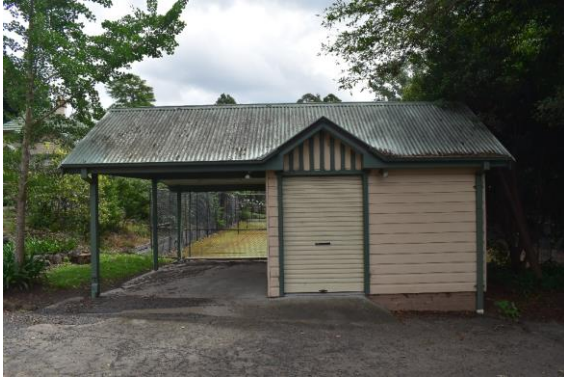
Figure 19. View north-east towards facade of c.1990s shed, showing corrugated iron roof with gable, weatherboard cladding and roller door.
