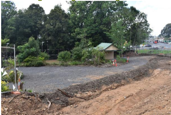
Figure 35. View from area of works towards driveway and c.1990s shed.
