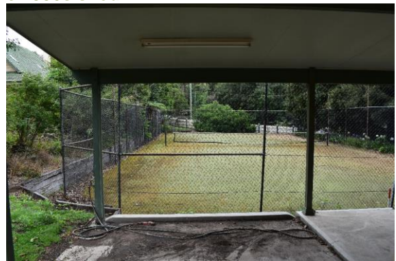
Figure 24. View north-east from c.1990s shed towards tennis courts and the former alignment of Brinawarr Street
