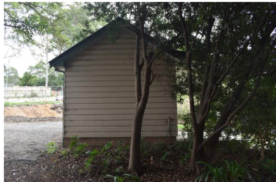
Figure 16. View of southern facade showing weatherboard cladding and tree coverage around c.1990s shed.
