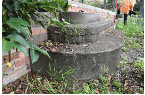
Figure 26. View of poured concrete steps on the north-eastern facade of c.1990s shed. The tennis courts are located immediately to the right.
