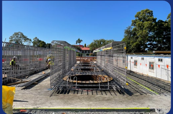
Steel reinforcement for the pile cap tubs
