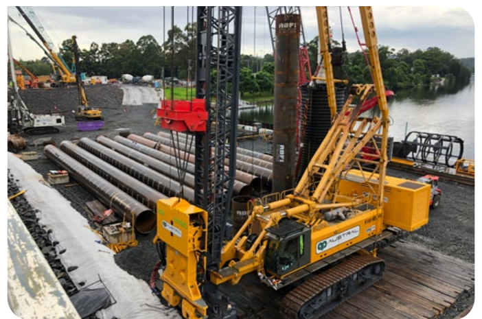
Pile casing being lifted into place
