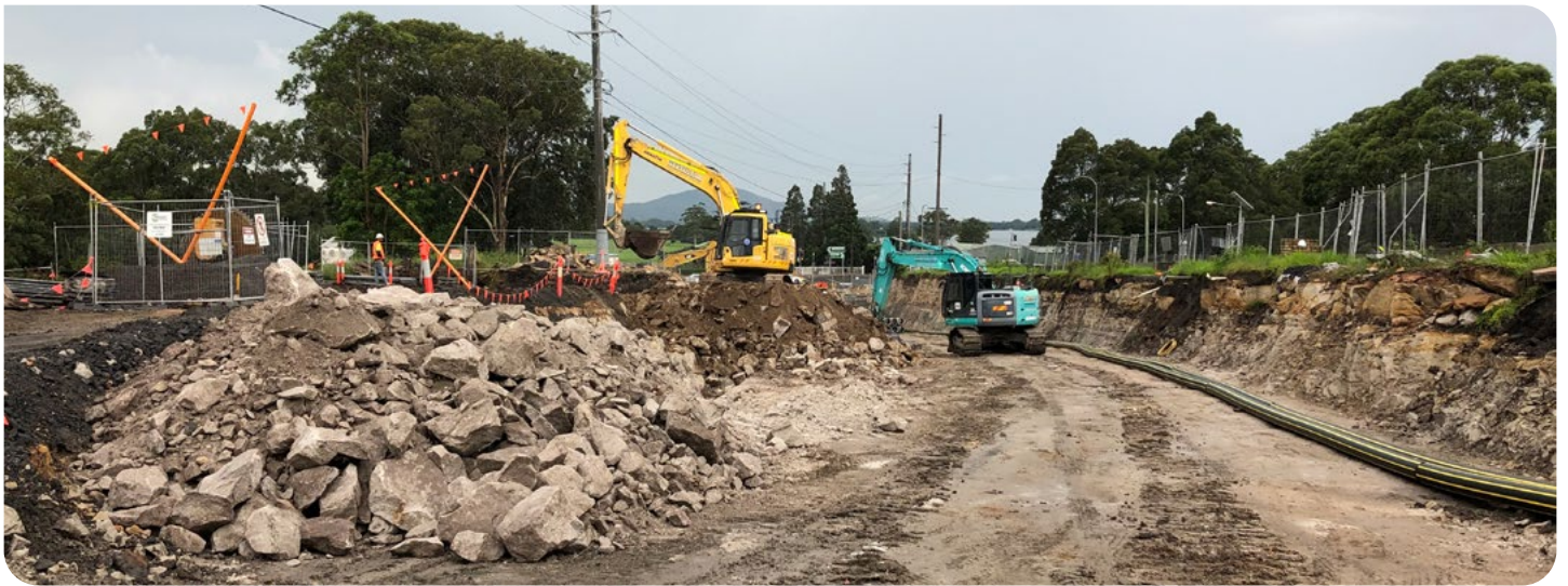
Material being removed from Illaroo Road
