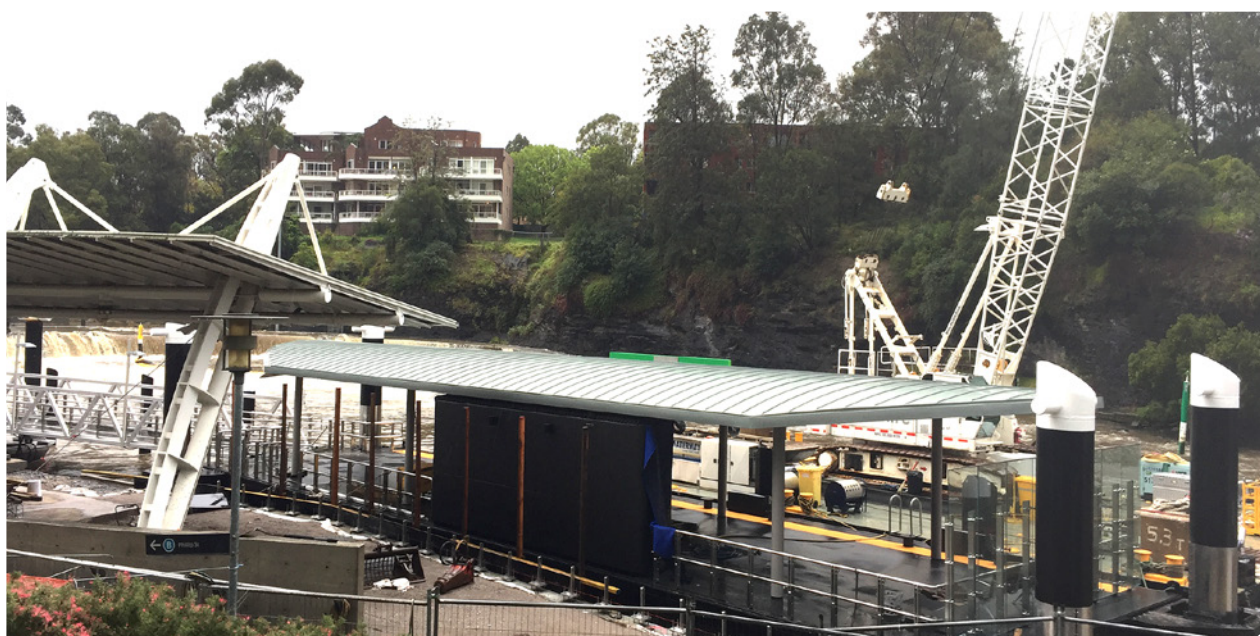
Parramatta Wharf construction nearing completion
