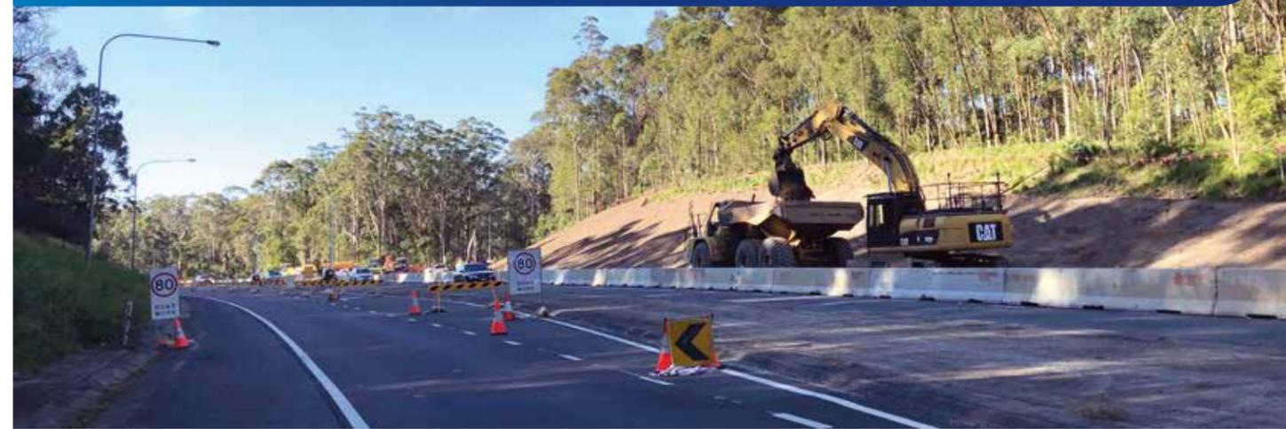
Construction of the Island Point Road roundabout is underway. The new roundabout at the intersection of the Princes Highway and Island Point Road in Tomerong will improve safety, traffic efficiency and connectivity around the Bay and Basin area.
