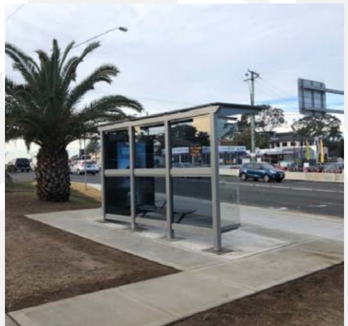
Relocated bus shelter at the new bus bay
