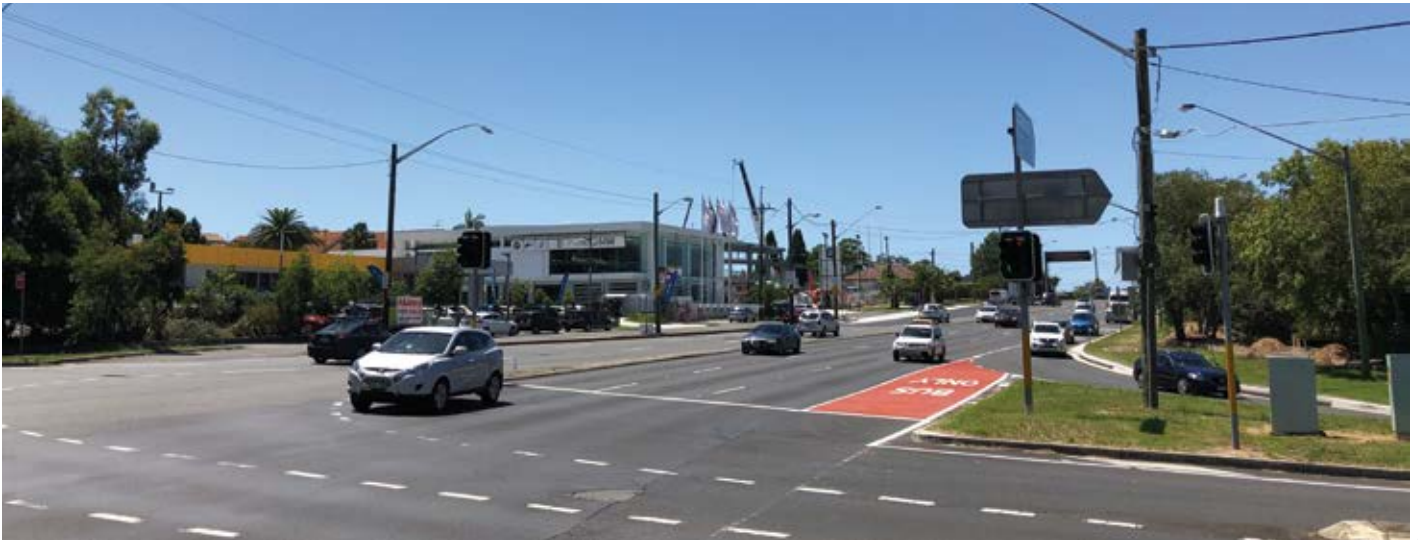
Recently-completed intersection work on Princes Highway and Port Hacking Road
